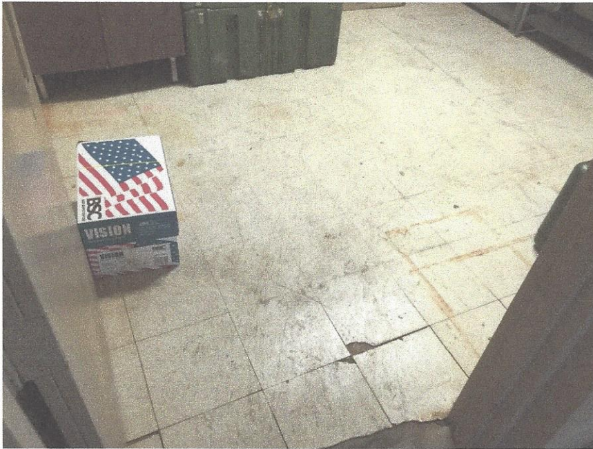
Mastic on floor tiles on Storage R&R (door 22)
