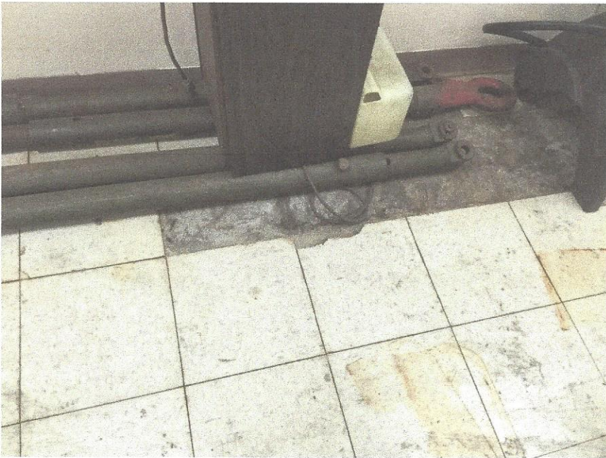
Mastic on floor tiles on Storage (door 21)
