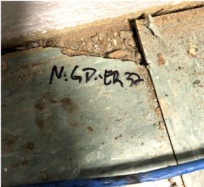
Asbestos Containing Green VFT 12"x 12" on top of VFT layer with Mastic Room 1-19
