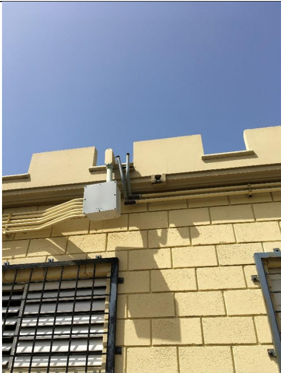
Photo #53: Ponce – PVC Electrical Condulet
