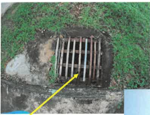
Remove and replace existing catch basin grate.
