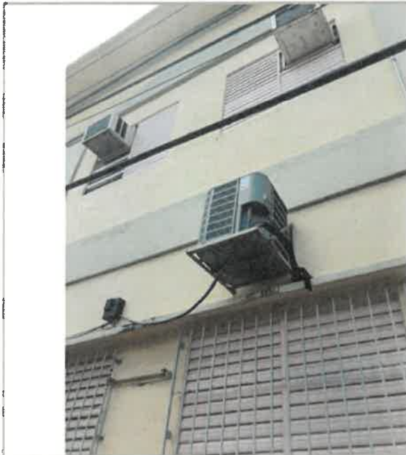
2nd Floor Health Certificate, 2 each of wall mounted 3 ton split A/C unit (view of the compressor), high winds, wind driven rain, wind blown debris and water intrusion damage the unit, 100% work completed (photo 2 of 3)
