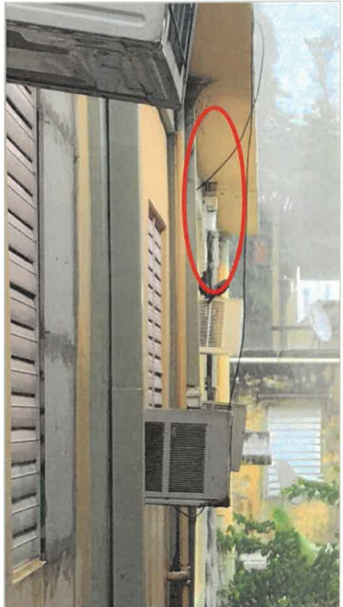
South Side Wall Exterior, metal 4in x 6in downspout, 90 LF long (view of another missing downspout and water falling profusely), high winds, wind driven rain, and wind blown debris blew off three 30ft long pieces, possible mitigation to effectively drain the south side of the building because all the roof drainage is on that side (where another building structure is erected just 5 ft apart) plus the emergency concrete stairs are on that side of the building, closing more that drainage area, 0% work completed (photo 3 of 3)
