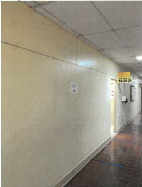
2nd Floor Main Hallway, 1,787 SF of Historic concrete wall paint, (119 + 119)ft x 86in high + (9ft x 9ft high), water intrusion through roof and window failure blistered and/or peeled off the paint, temporarily painted, 0% work completed
