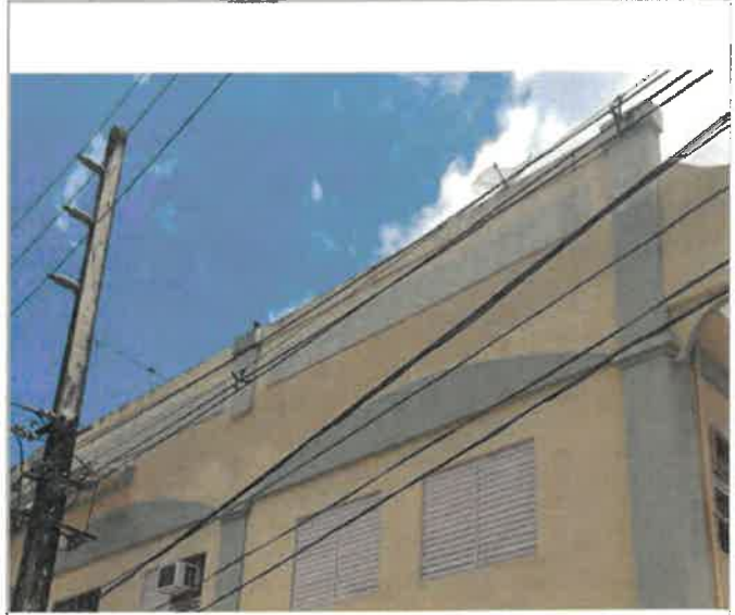
West Side Wall Building Exterior, 3 CY of Historic concrete cornice and paint, 40 FT long x 30 IN wide x 8 IN high, high winds, wind driven rain, and wind blown debris broke and/or loosened the cornice, it was demolished by Applicant, 0% work completed (photo 2 of 2)
