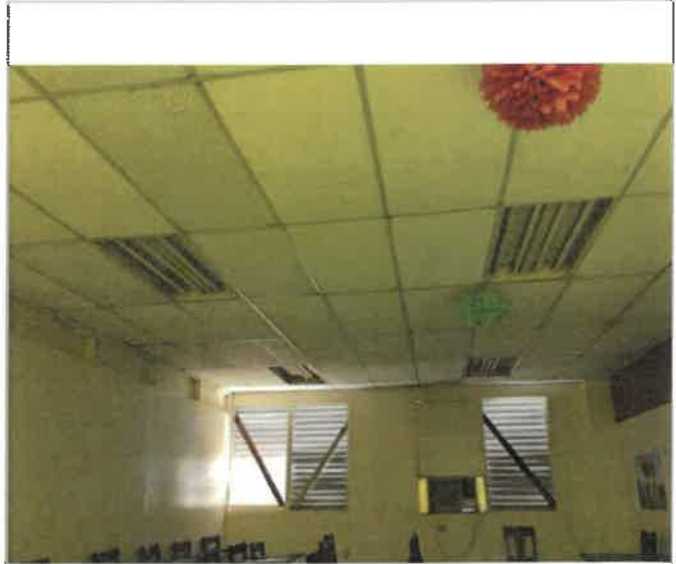
2nd Floor Conference Room 1, suspended lay-in acoustic 2 x 4 ceiling tile; fluorescent 2 x 4 drop-in ceiling light fixture, 4 tubes; and wall paint, water intrusion through roof and window failure damaged the area, 0% work completed
