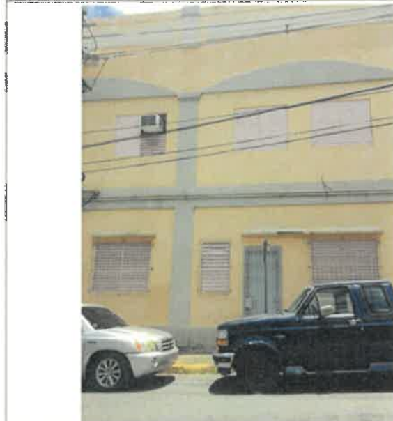
Building Exterior, aluminum jalousie window sealing to concrete, 1,054 LF long, 43 windows (6ft x 5ft) + 5 windows (3ft x 5ft) + 2 windows (5ft x 2ft), high winds, wind driven rain, and wind blown debris damage the seal, 0% work completed (photo 2 of 2)
