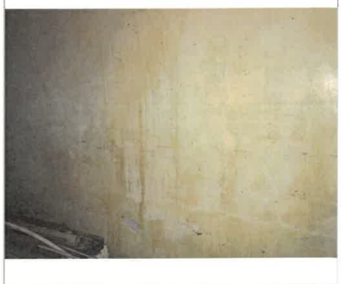
1st Floor Storage Room next to Serology, 470 SF of concrete wall paint, 54.75 LF long x 8.58 FT high, water intrusion through window failure, surface water flooding, and prolonged humidity blistered and/or peeled off the paint, 0% work completed (photo 2 of 2)
