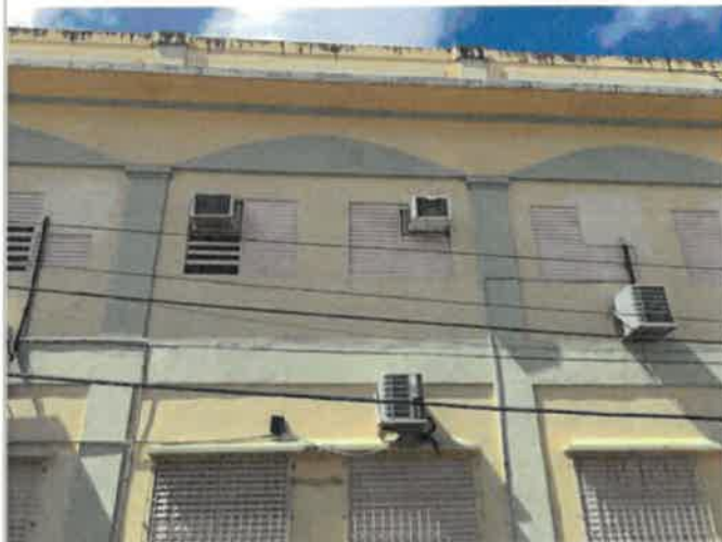
Building Exterior, aluminum jalousie window sealing to concrete, 1,054 LF long, 43 windows (6ft x 5ft) + 5 windows (3ft x 5ft) + 2 windows (5ft x 2ft), high winds, wind driven rain, and wind blown debris damage the seal, 0% work completed (photo 1 of 2)
