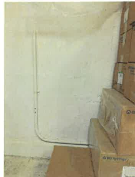
1st Floor Storage Room, 405 SF of Historic concrete wall paint, 45 FT long x 9 FT high, water intrusion through window failure and surface water flooding blistered and/or peeled off the paint, 0% work completed (photo 1 of 3)
