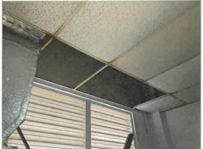
1st Floor Storage Room, 270 SF of suspended lay-in acoustic 2 x 4 ceiling tile, 45 FT long x 6 FT wide, the first two rows next to the outside wall, water intrusion through window failure damage the tile, 0% work completed (photo 2 of 2)
