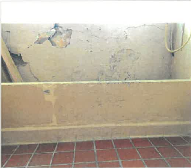
2nd Floor Restrooms Hallway, 32 SF of Historic concrete wall plaster, 8 FT long x 4 FT high, water intrusion through roof and window failure detached and/or scraped the plaster under the window opening, 0% work completed
