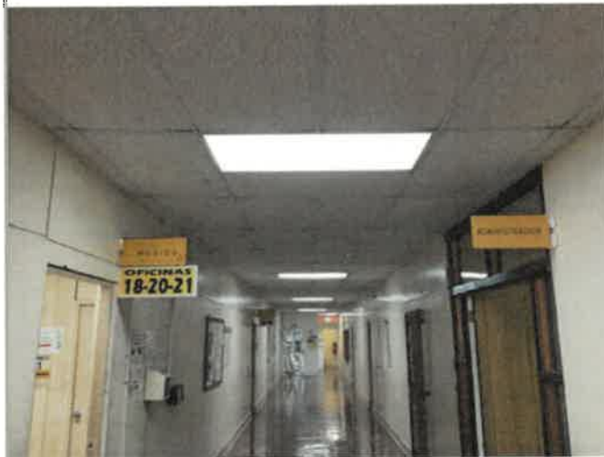
2nd Floor Main Hallway, 6 each of fluorescent drop-in ceiling light fixture, 4 tubes, 2 FT long x 4 FT wide, water intrusion through roof and window failure damage the fixture, the tubes were replaced with LED, 0% work completed
