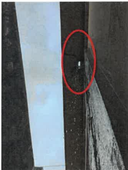
South Side Wall Exterior, metal 4in x 6in downspout, 90 LF long (view of an opening on the roof where the downspout was), wind driven rain, and wind blown debris blew off three 30ft long pieces, 0% work completed (photo 2 of 3)
