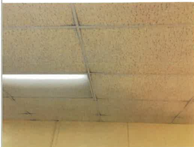
2nd Floor Finances, 448 SF of suspended lay-in acoustic 2 x 4 ceiling tile, 32 FT long x 14 FT wide, temporarily replaced, and 4 each of fluorescent drop-in ceiling light fixture, 4 tubes, 2 FT long x 4 FT wide, water intrusion through roof and window failure damage the fixture, 0% work completed
