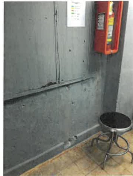
1st Floor Clinical Laboratory, 416 SF of Historic concrete wall paint, 52 LF long x 8 FT high, water intrusion through window failure blistered, and/or peeled off the paint, temporarily painted, 0% work completed (photo 1 of 2)
