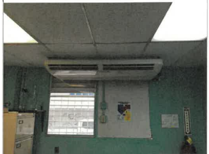
1st Floor Clinical Laboratory, 1 each of wall mounted AirMax CCF4-60CR 5 ton split A/C unit repairs, high winds, wind driven rain, wind blown debris and water intrusion damage the unit, 100% work completed (photo 1 of 2)
