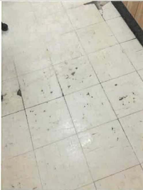
1st Floor Tuberculin Results Reading, 80 SF of vinyl composition tile (VCT) flooring, 12 FT long x 6.67 FT wide, surface water flooding, and prolonged humidity detached, lifted and stained the tiles, ongoing problem, 0% work completed (photo 2 of 2)
