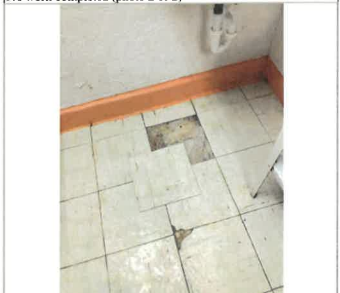
1st Floor Tuberculin Results Reading, 80 SF of vinyl composition tile (VCT) flooring, 12 FT long x 6.67 FT wide, surface water flooding, and prolonged humidity detached, lifted and stained the tiles, ongoing problem, 0% work completed (photo 1 of 2)
