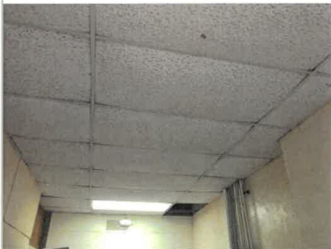
2nd Floor Restrooms Hallway, 288 SF of suspended lay-in acoustic 2 x 4 ceiling tile, 36 FT long x 8 FT wide, water intrusion through roof and window failure damage the tile, temporarily replaced, 0% work completed
