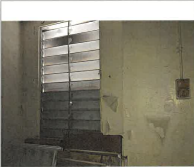
1st Floor Maintenance Storage Area, 815 SF of Historic concrete wall paint, 90.5 LF long x 9 FT high, water intrusion through window failure blistered and/or peeled off the paint, 0% work completed
