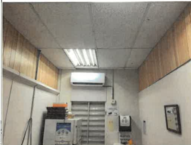
1st Floor Tuberculin Results Reading, 1 each of window mounted 12,000 BTU A/C unit, high winds, wind driven rain, wind blown debris and water intrusion damage the unit, replaced with Air-Con AEDEM4C4512 split unit, 100% work completed (photo 1 of 2)
