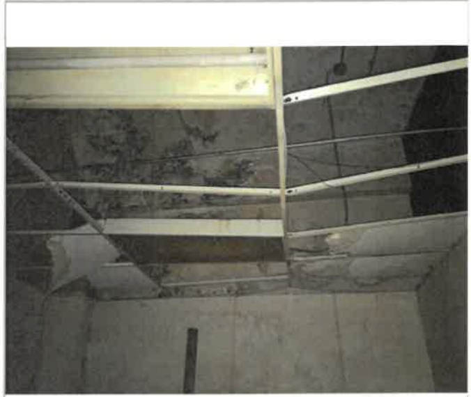
1st Floor Maintenance Storage Area, 544 SF of suspended lay-in acoustic 2 x 4 ceiling tile, the first three rows next to the outside wall (this is a corner area) (64ft x 6ft) + (20ft x 8ft), water intrusion through window failure damage the tile, 0% work completed
