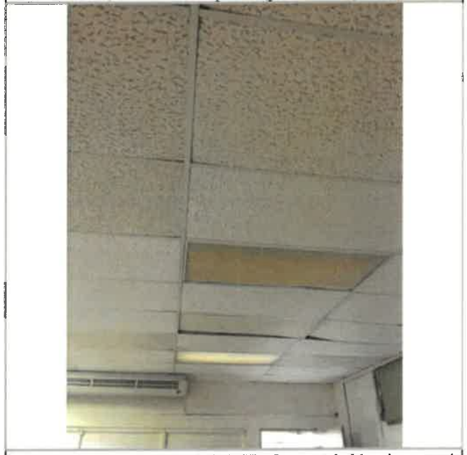
2nd Floor Administration, 1,829 SF of suspended lay-in acoustic 2 x 4 ceiling tile, 59 FT long x 31 FT wide, water intrusion through roof failure damage the tile. 0% work completed (photo 1 of 2)
