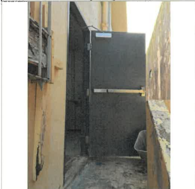
South Side Wall Exterior, 1 each of wooden security door. 3 FT wide x 7 FT high, high winds and wind blown debris broke the door, was replaced with a metal security door, 100% work completed
