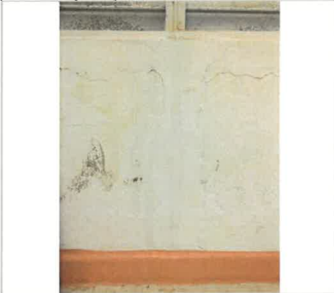
1st Floor Tuberculin Results Reading, 60 SF of Historic concrete wall paint, 6.67 FT long x 9 FT high, water intrusion through window failure and surface water flooding from water accumulated between the affected and the adjacent buildings blistered and/or peeled off the paint, ongoing problem, temporarily painted, 0% work completed
