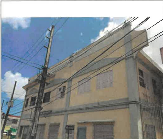
West Side Wall Building Exterior, 3 CY of Historic concrete cornice and paint, 40 FT long x 30 IN wide x 8 IN high, high winds, wind driven rain, and wind blown debris broke and/or loosened the cornice, it was demolished by Applicant, 0% work completed (photo 1 of 2)
