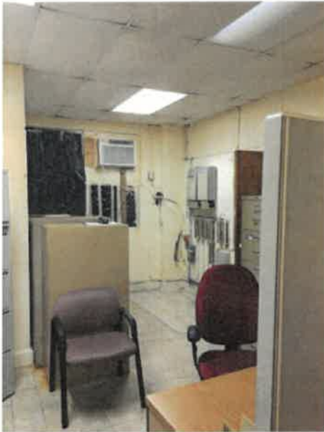
2nd Floor Finance, suspended lay-in acoustic 2 x 4 ceiling tile, temporarily replaced, fluorescent 2 x 4 drop-in ceiling light fixtures, and wall paint, all temporarily fixed, 0% work completed
