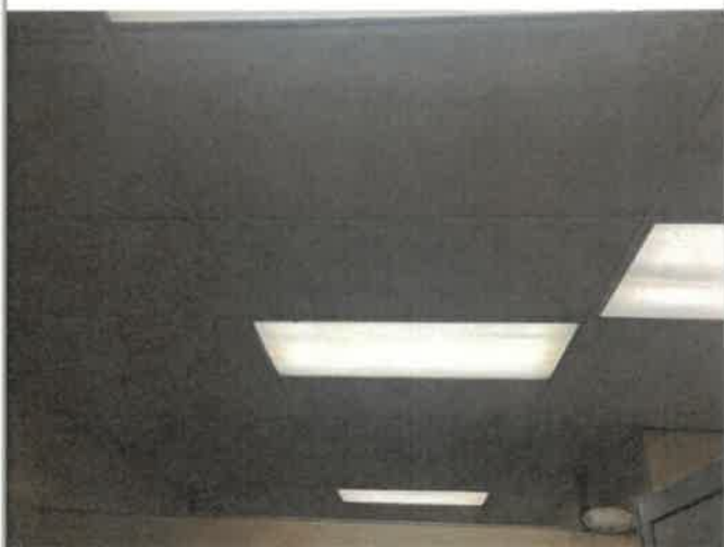
2nd Floor Epidemiology, 704 SF of suspended lay-in acoustic 2 x 4 ceiling tile, 22 FT long x 32 FT wide, and 7 each of fluorescent drop-in ceiling light fixture, 4 tubes, 2 FT long x 4 FT wide, water intrusion through roof and window failure damage the fixture and tiles, temporarily replaced tiles and tubes, 0% work completed
