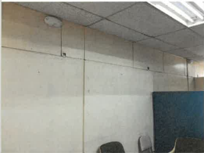
2nd Floor Doctor, Social Work and Mother & Child, 518 SF of Historic concrete wall paint, and 56 SF of wooden panel wall paint, water intrusion through roof and window failure blistered and/or peeled off the paint, temporarily painted, 0% work completed
