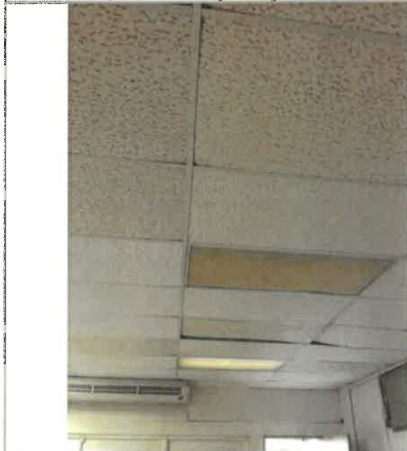
2nd Floor Administration, 1,829 SF of suspended lay-in acoustic 2 x 4 ceiling tile, 59 FT long x 31 FT wide, water intrusion through roof failure damage the tile, 0% work completed (photo 1 of 2)
