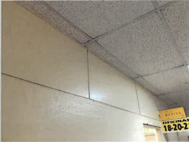
2nd Floor Main Hallway, 455 SF of wooden panel wall paint, 260 LF long x 21 IN high, water intrusion through roof and window failure blistered and/or peeled off the paint, temporarily painted, 0% work completed (photo 1 of 2)
