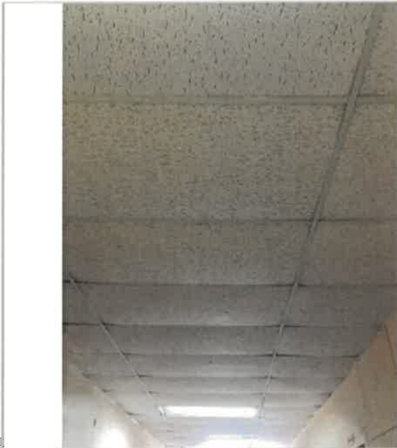
2nd Floor Main Hallway, 1,071 SF of suspended lay-in acoustic 2 x 4 ceiling tile, 119 FT long x 9 FT wide, water intrusion through roof failure damage the tile, temporarily replaced, 0% work completed
