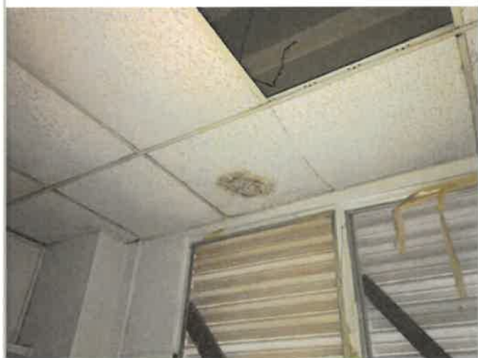
1st Floor Storage Room, 270 SF of suspended lay-in acoustic 2 x 4 ceiling tile, 45 FT long x 6 FT wide, the first two rows next to the outside wall, water intrusion through window failure damage the tile, 0% work completed (photo 1 of 2)
