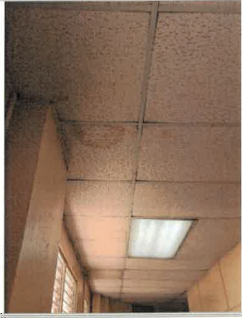
2nd Floor Stairs Hallway, 132 SF of suspended lay-in acoustic 2 x 4 ceiling tile, 22 FT long x 6 FT wide, water intrusion through roof failure damage the tile, temporarily replaced, 0% work completed
