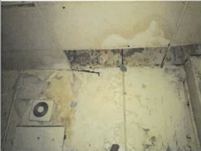
1st Floor Lunch Area, 162 SF of Historic concrete wall paint, 18 FT long x 9 FT high, and 144 SF of suspended lay-in acoustic 2 x 4 ceiling tile, 18 FT long x 8 FT wide, the first two rows next to the outside wall, excessive humidity caused damage, 0% work completed
