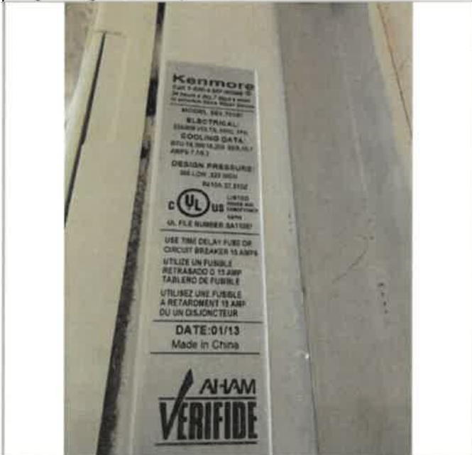
2nd Floor Administration, 1 each of window mounted 18,500 BTU A/C unit, Kenmore 253.70181, high winds, wind driven rain, wind blown debris, power surges, and water intrusion damage the unit, 0% work completed (photo 2 of 2)
