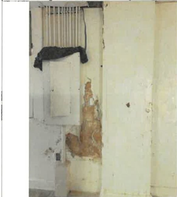
2nd Floor Administration, 160 SF of Historic concrete wall plaster and paint, 20 FT long x 8 FT high, water intrusion through roof and window failure, and water cascading down the outside side of the wall because of a missing downspout detached and scraped the plaster, 0% work completed
