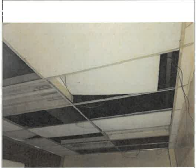
2nd Floor Doctor, Social Work and Mother & Child, 2 x 4 fluorescent drop-in ceiling light fixture, 4 tubes, and suspended acoustic ceiling tiles, water intrusion through roof and window failure damaged the fixtures, (photo 3 of 3)
