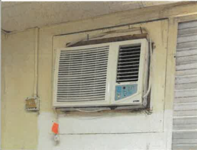
2nd Floor Finances, Epidemiology and Vaccination, 1 each (for each room) of window mounted 18,500 BTU A/C unit, high winds, wind driven rain, wind blown debris and water intrusion damage the units, 0% work completed
