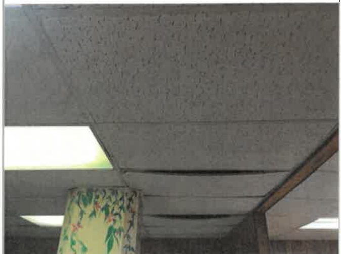
1st Floor Billing, 110 SF of suspended lay-in acoustic 2 x 4 ceiling tile, 22 FT long x 5 FT wide, the first two rows next to the outside wall, water intrusion through window failure damage the tile, 0% work completed
