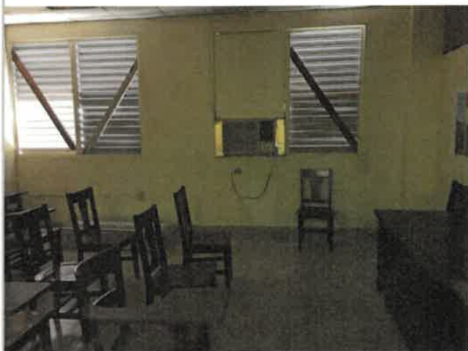
2nd Floor Conference Room 1, 497 SF of Historic concrete wall paint, side walls (31 + 17)ft x 86 in high + outside wall (17ft x 9ft high), water intrusion through roof and window failure blistered and/or peeled off the paint, temporarily painted, 0% work completed
