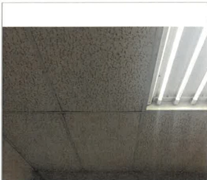
2nd Floor Vaccination, 12 each of fluorescent drop-in ceiling light fixture, 4 tubes, 2 FT long x 4 FT wide, and 720 SF of suspended lay-in acoustic 2 x 4 ceiling tile, 36 FT long x 20 FT wide, water intrusion through roof and window failure damage the tile and fixtures, temporarily replaced tiles and tubes
