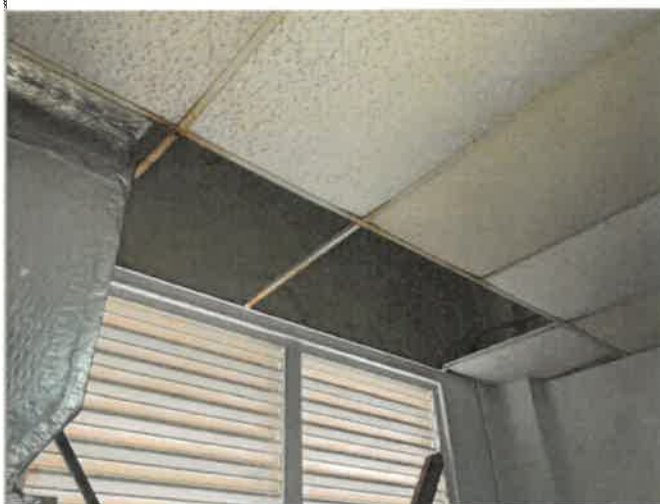
1st Floor Storage Room, 270 SF of suspended lay-in acoustic 2 x 4 ceiling tile, 45 FT long x 6 FT wide, the first two rows next to the outside wall, water intrusion through window failure damage the tile, 0% work completed (photo 2 of 2)
