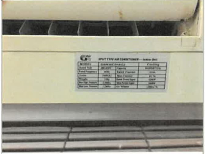
2nd Floor Health Certificate, 2 each of wall mounted 3 ton split A/C unit (blower specifications), high winds, wind driven rain, wind blown debris and water intrusion damage the unit, 100% work completed (photo 1 of 3)
