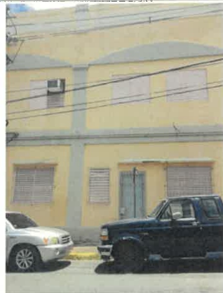
Building Exterior, aluminum jalousie window sealing to concrete, 1,054 LF long, 43 windows (6ft x 5ft) + 5 windows (3ft x 5ft) + 2 windows (5ft x 2ft), high winds, wind driven rain, and wind blown debris damage the seal, 0% work completed (photo 2 of 2)
