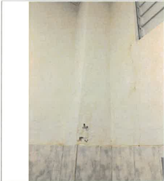
1st Floor Men's Restroom, 54 SF of Historic concrete wall paint, 9.5 FT long x 5.67 FT high, there are glazed tiles on the lower part of the wall, water intrusion through window failure blistered and/or peeled off the paint, ongoing problem, 0% work completed
