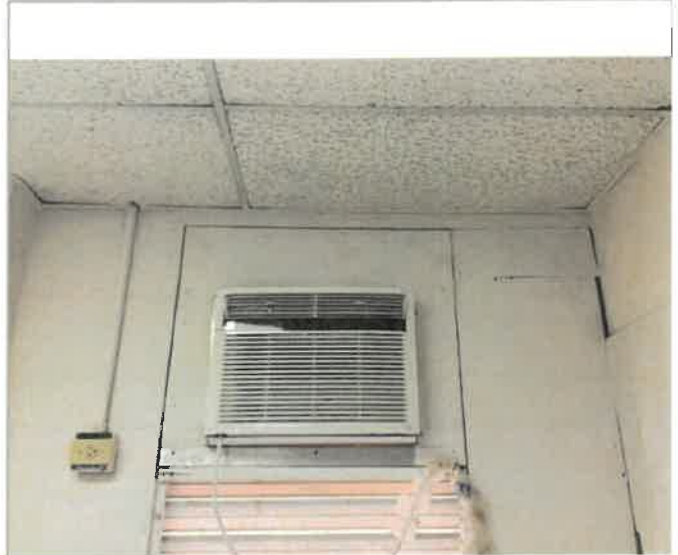
2nd Floor Administration, 1 each of window mounted 18,500 BTU A/C unit, Kenmore 253.70181, high winds, wind driven rain, wind blown debris, power surges, and water intrusion damage the unit, 0% work completed (photo 1 of 2)
