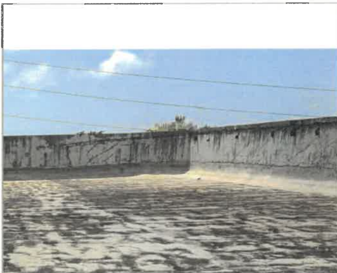
Roof Parapet, 1,960 SF of parapet wall paint, 280 LF long x 7 FT high, high winds, wind driven rain, and wind blown debris blistered and peeled off the paint, 0% work completed
