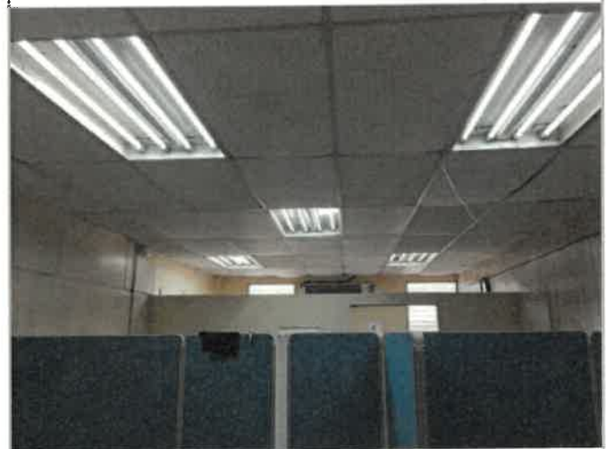
2nd Floor Doctor, Social Work and Mother & Child, 2 x 4 fluorescent drop-in ceiling light fixture, 4 tubes, and suspended acoustic ceiling tiles, water intrusion through roof and window failure damaged the fixtures, the tubes were replaced with LED types, (photo 1 of 3)
