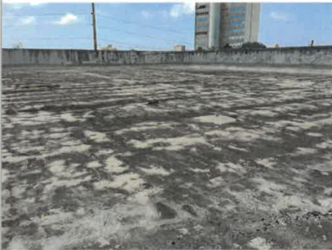
Roof, 9,600 SF of built-up membrane roof waterproofing treatment, 120 FT long x 80 FT wide, high winds, wind driven rain, and wind blown debris detached, bubbled, and peeled off the treatment, 0% work completed (photo 1 of 2)
