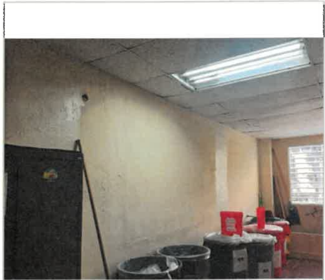
2nd Floor Restrooms Hallway, 720 SF of Historic concrete wall paint, 80 LF long x 9 FT high, water intrusion through roof and window failure blistered and/or peeled off the paint, temporarily painted, 0% work completed
