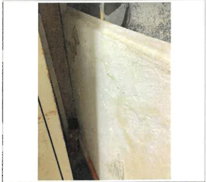
1st Floor Serology, 219 SF of Historic concrete wall paint, 24.25 FT long x 9 FT high, water intrusion through window failure and surface water flooding from water accumulated between the affected and the adjacent buildings blistered and/or peeled off the paint, ongoing problem, temporarily painted, 0% work completed (photo 2 of 2)
