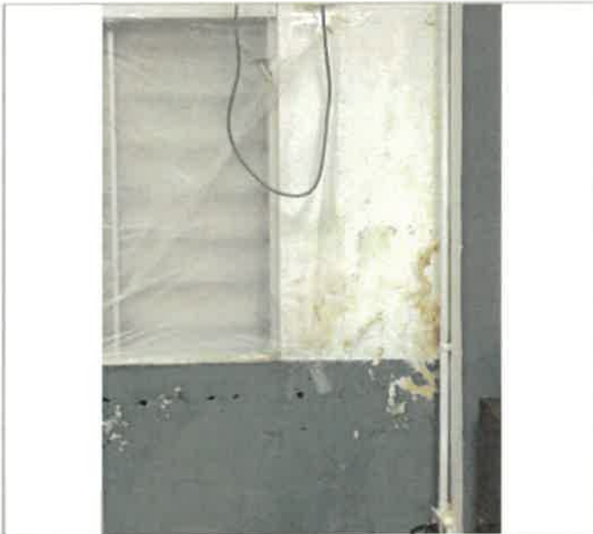
1st Floor Serology, 219 SF of Historic concrete wall paint, 24.25 FT long x 9 FT high, water intrusion through window failure and surface water flooding from water accumulated between the affected and the adjacent buildings blistered and/or peeled off the paint, ongoing problem, temporarily painted, 0% work completed (photo 1 of 2)
