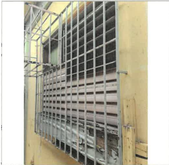
South Side Wall Exterior, 6 each of aluminum jalousie window, 5 FT long x 3 FT wide, high winds and wind blown debris broke and/or bent the windows, should be verified for Historic characteristics. 0% work completed (photo 1 of 2)
