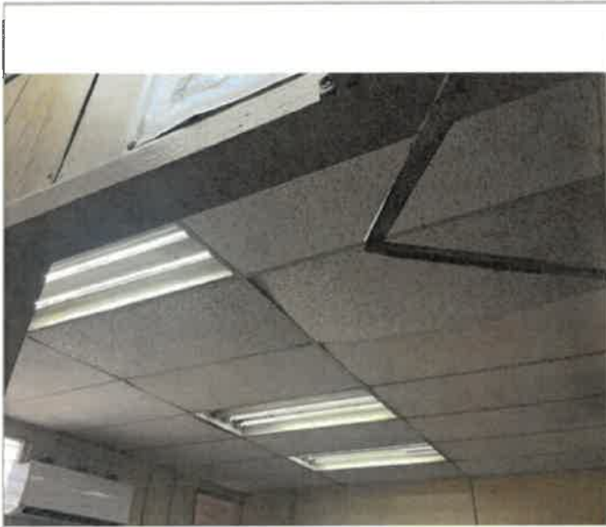
2nd Floor Doctor, Social Work and Mother & Child, 2 x 4 fluorescent drop-in ceiling light fixture, 4 tubes, and suspended acoustic ceiling tiles, water intrusion through roof and window failure damaged the fixtures, the tubes were replaced with LED types, (photo 2 of 3)
