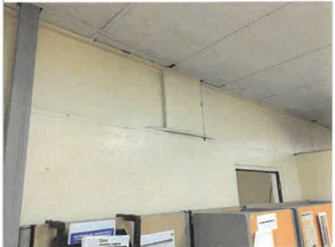
2nd Floor Epidemiology, 657 SF of Historic concrete wall paint, (22ft x 9ft high) + 2 walls of (32ft x 86in high), and 112 SF of wooden panel wall paint, 64 LF long x 21 IN high, 2 walls of (32ft x 21in high), water intrusion through roof and window failure blistered and/or peeled off the paint, temporarily painted, 0% work completed
