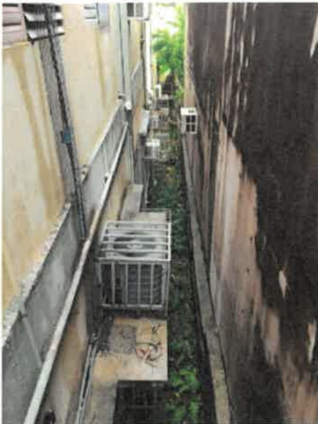
South Side Wall Exterior, view of the narrow space between the affected building and the adjacent building, which serves as the roof water drainage area to the outside of the property, possible mitigation (photo 1 of 3)
