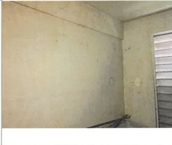
1st Floor Storage Room next to Serology, 470 SF of concrete wall paint, 54.75 LF long x 8.58 FT high, water intrusion through window failure, surface water flooding, and prolonged humidity blistered and/or peeled off the paint, 0% work completed (photo 1 of 2)
