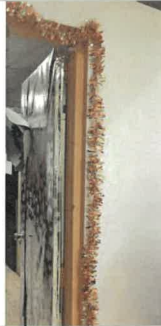
2nd Floor Vaccination, 309 SF of Historic concrete wall paint, (20ft x 9ft high) + (18ft x 86in high), water intrusion through roof and window failure blistered and/or peeled off the paint, temporarily painted, 0% work completed
