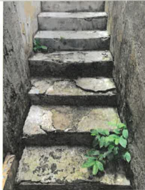
South Side Wall Exterior, 28 SF of Historic concrete stairs plaster and paint, 32 IN long x 12 IN wide x 6 IN high, 7 steps, eroded by falling water directly from the roof because of a blown off downspout, 0% work completed (photo 1 of 2)
