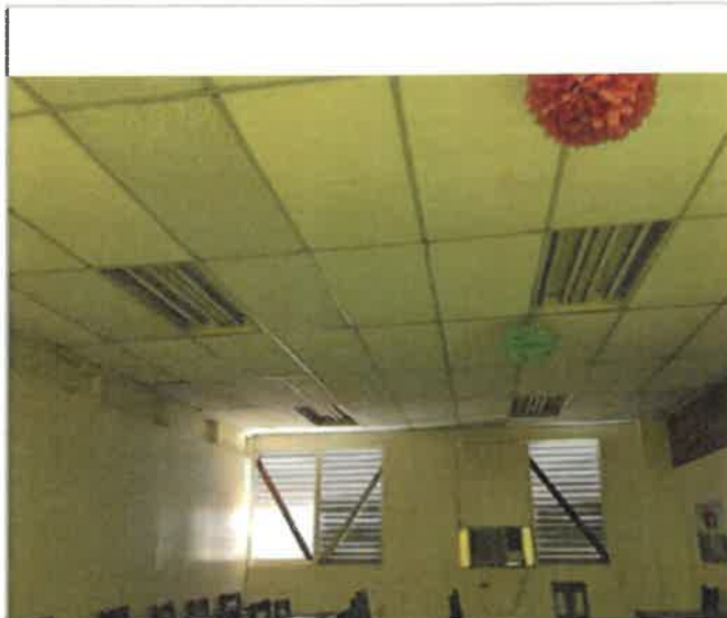
2nd Floor Conference Room 1, suspended lay-in acoustic 2 x 4 ceiling tile; fluorescent 2 x 4 drop-in ceiling light fixture, 4 tubes; and wall paint, water intrusion through roof and window failure damaged the area, 0% work completed
