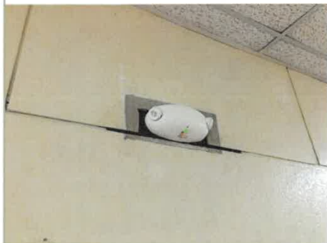
2nd Floor Hallways and Offices, 7 each of wall mounted Lithonia Emergency light fixture, 2 lamps, view of the new ones, water intrusion through roof and window failure damaged the fixtures, 100% work completed (photo 2 of 3)
