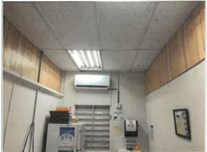
1st Floor Tuberculin Results Reading, 1 each of window mounted 12,000 BTU A/C unit, high winds, wind driven rain, wind blown debris and water intrusion damage the unit, replaced with Air-Con AEDM4C4512 split unit, 100% work completed (photo 1 of 2)
