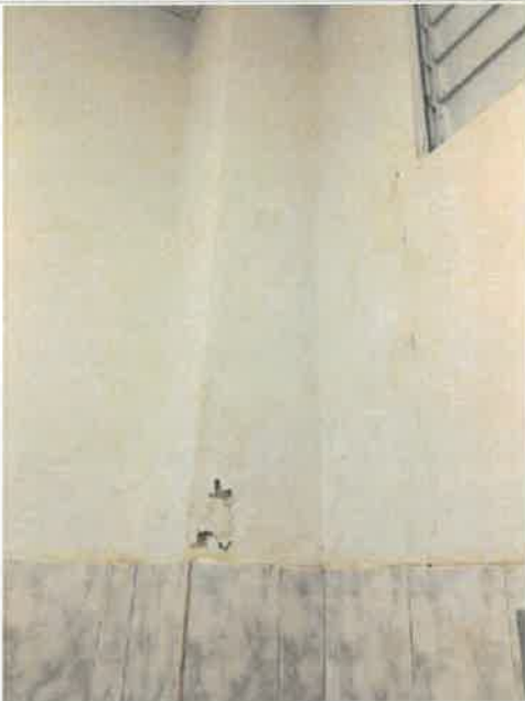
1st Floor Men's Restroom, 54 SF of Historic concrete wall paint, 9.5 FT long x 5.67 FT high, there are glazed tiles on the lower part of the wall, water intrusion through window failure blistered and/or peeled off the paint, ongoing problem, 0% work completed
