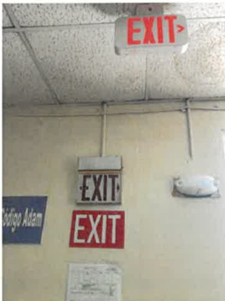
2nd Floor Main Hallway, 1 each of suspended ceiling mounted Exit light fixture, water intrusion through roof and window failure damaged the fixtures, 100% work complete
