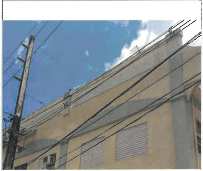
West Side Wall Building Exterior, 3 CY of Historic concrete cornice and paint, 40 FT long x 30 IN wide x 8 IN high, high winds, wind driven rain, and wind blown debris broke and/or loosened the cornice, it was demolished by Applicant, 0% work completed (photo 2 of 2)
