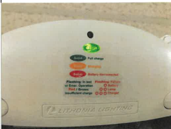
2nd Floor Hallways and Offices, 7 each of wall mounted Lithonia Emergency light fixture, 2 lamps, view of the new ones, water intrusion through roof and window failure damaged the fixtures, 100% work completed (photo 3 of 3)
