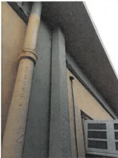
South Side Wall Exterior, metal 4in x 6in downspout, 90 LF long (view of an undamaged one), high winds, wind driven rain, and wind blown debris blew off three 30ft long pieces, possible mitigation to effectively drain the south side of the building because all the roof drainage is on that side (where another building structure is erected just 5 ft apart) plus the emergency concrete stairs are on that side of the building, closing more that drainage area, 0% work completed (photo 1 of 3)
