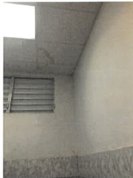
1st Floor Men's Restroom, 48 SF of suspended lay-in acoustic 2 x 4 ceiling tile, 9.5 FT long x 5 FT wide, the first two rows next to the outside wall, water intrusion through window failure damage the tile, ongoing problem, 0% work completed
