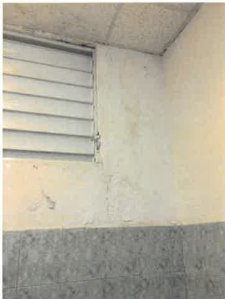
1st Floor Women's Restroom, 35 SF of Historic concrete wall paint, 8.67 FT long x 4 FT high, there are glazed tiles on the lower part of the wall, water intrusion through window failure blistered and/or peeled off the paint, 0% work complete
