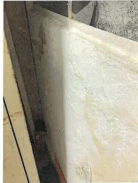
1st Floor Serology, 219 SF of Historic concrete wall paint, 24.25 FT long x 9 FT high, water intrusion through window failure and surface water flooding from water accumulated between the affected and the adjacent buildings blistered and/or peeled off the paint, ongoing problem, temporarily painted, 0% work completed (photo 2 of 2)
