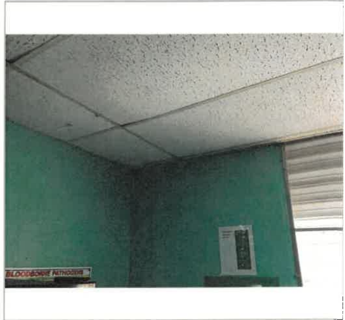
1st Floor Clinical Laboratory, 256 SF of suspended lay-in acoustic 2 x 4 ceiling tile, the first two rows next to the outside wall (this is a corner area) (8ft x 20ft) + (4ft x 24ft), water intrusion through window failure damage the tile, temporarily replaced, 0% work completed
