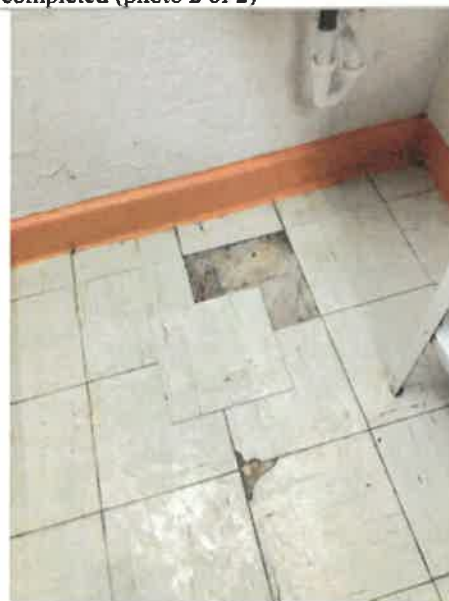
1st Floor Tuberculin Results Reading, 80 SF of vinyl composition tile (VCT) flooring, 12 FT long x 6.67 FT wide, surface water flooding, and prolonged humidity detached, lifted and stained the tiles, ongoing problem, 0% work completed (photo 1 of 2)
