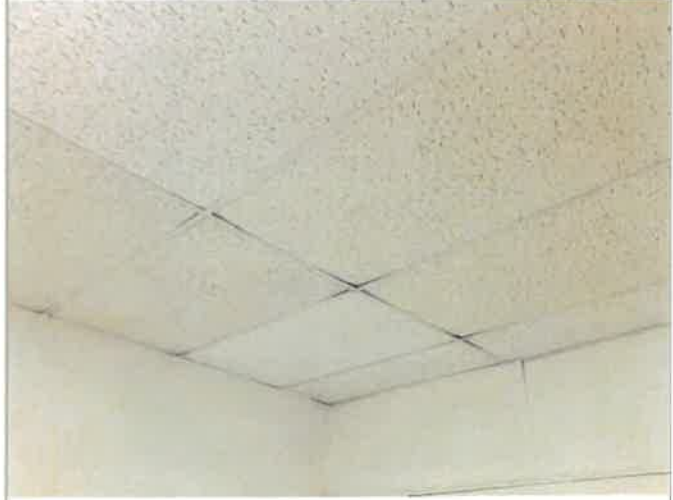
2nd Floor Health Certificate, 448 SF of suspended lay-in acoustic 2 x 4 ceiling tile, 32 FT long x 14 FT wide, water intrusion through roof and window failure damage the tile, temporarily replaced, 0% work completed
