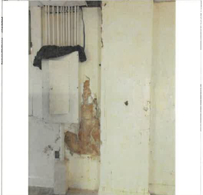
2nd Floor Administration, 160 SF of Historic concrete wall plaster and paint, 20 FT long x 8 FT high. water intrusion through roof and window failure, and water cascading down the outside side of the wall because of a missing downspout detached and scraped the plaster, 0% work completed
