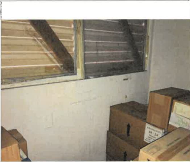
1st Floor Storage Room, 405 SF of Historic concrete wall paint, 45 FT long x 9 FT high, water intrusion through window failure and surface water flooding blistered and/or peeled off the paint, 0% work completed (photo 2 of 3)
