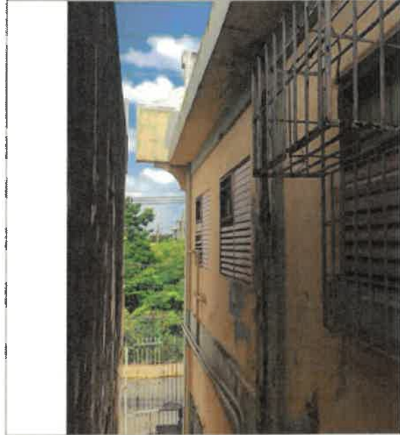
South Side Wall Exterior, 6 each of aluminum jalousie window, 5 FT long x 3 FT wide, high winds and wind blown debris broke and/or bent the windows, should be verified for Historic characteristics, 0% work completed (photo 2 of 2)
