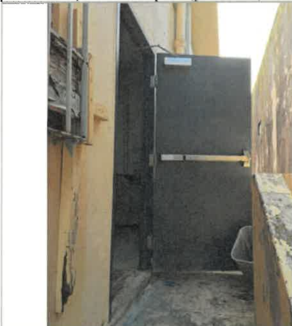
South Side Wall Exterior, 1 each of wooden security door, 3 FT wide x 7 FT high, high winds and wind blown debris broke the door, was replaced with a metal security door, 100% work completed
