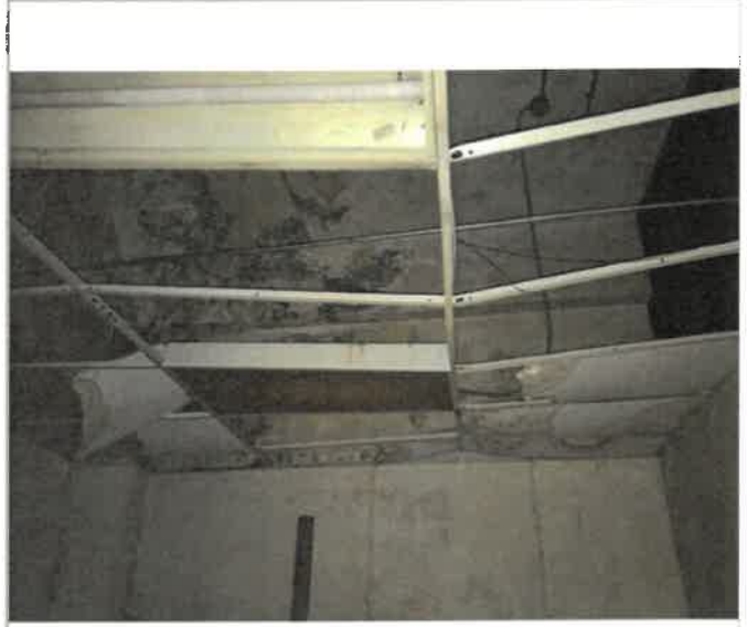
1st Floor Maintenance Storage Area, 544 SF of suspended lay-in acoustic 2 x 4 ceiling tile, the first three rows next to the outside wall (this is a corner area) (64ft x 6ft) + (20ft x 8ft), water intrusion through window failure damage the tile, 0% work completed
