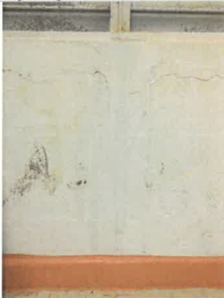
1st Floor Tuberculin Results Reading, 60 SF of Historic concrete wall paint, 6.67 FT long x 9 FT high, water intrusion through window failure and surface water flooding from water accumulated between the affected and the adjacent buildings blistered and/or peeled off the paint, ongoing problem, temporarily painted, 0% work completed
