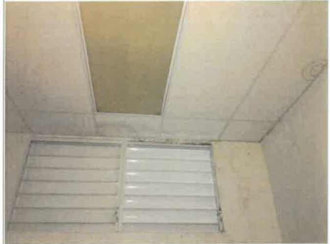
1st Floor Women's Restroom, 44 SF of suspended lay-in acoustic 2 x 4 ceiling tile, 8.67 FT long x 5 FT wide, the first two rows next to the outside wall, water intrusion through window failure damage the tile, ongoing problem, 0% work complete
