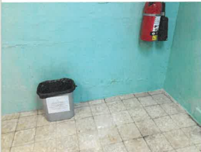
1st Floor Clinical Laboratory, 416 SF of Historic concrete wall paint, 52 LF long x 8 FT high, water intrusion through window failure blistered, and/or peeled off the paint, temporarily painted, 0% work completed (photo 2 of 2)
