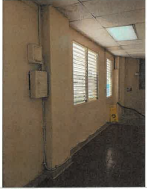
2nd Floor Stairs Hallway, 356 SF of Historic concrete wall paint, (22ft x 86 in high) + (22ft x 9ft high), water intrusion through roof and window failure blistered and/or peeled off the paint, temporarily painted, 0% work completed
