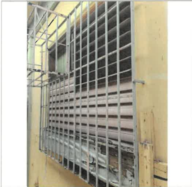
South Side Wall Exterior, 6 each of aluminum jalousie window, 5 FT long x 3 FT wide, high winds and wind blown debris broke and/or bent the windows, should be verified for Historic characteristics, 0% work completed (photo 1 of 2)
