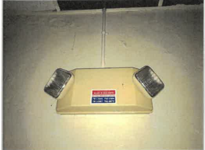
2nd Floor Hallways and Offices, 7 each of wall mounted Lithonia Emergency light fixture, 2 lamps, water intrusion through roof and window failure damaged the fixtures, 100% work completed (photo 1 of 3)
