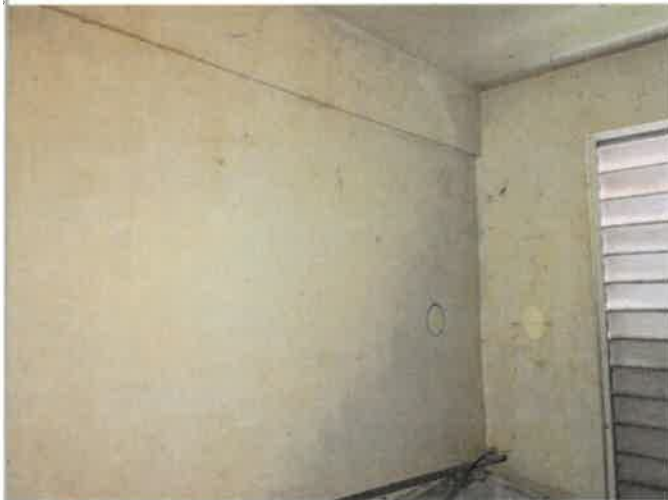
1st Floor Storage Room next to Serology, 470 SF of concrete wall paint, 54.75 LF long x 8.58 FT high, water intrusion through window failure, surface water flooding, and prolonged humidity blistered and/or peeled off the paint, 0% work completed (photo 1 of 2)
