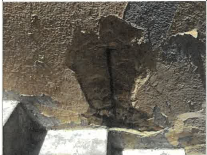
South Side Wall Exterior, 6 SF of Historic concrete sidewalk plaster and paint, 2 FT long x 3 FT wide, eroded by falling water from the roof because of a blown off downspout, 0% work completed
