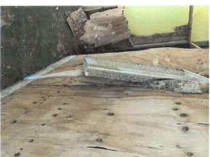
4- The contractor must include the repair of existing damaged security grate sections (40 SF Approx.)
