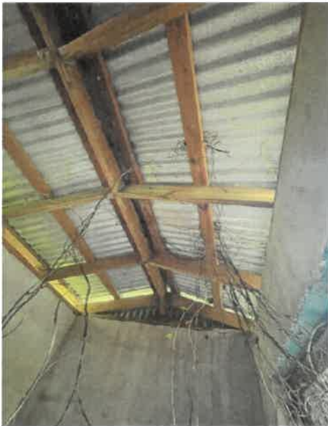
Photo 4: Existing Pump House
