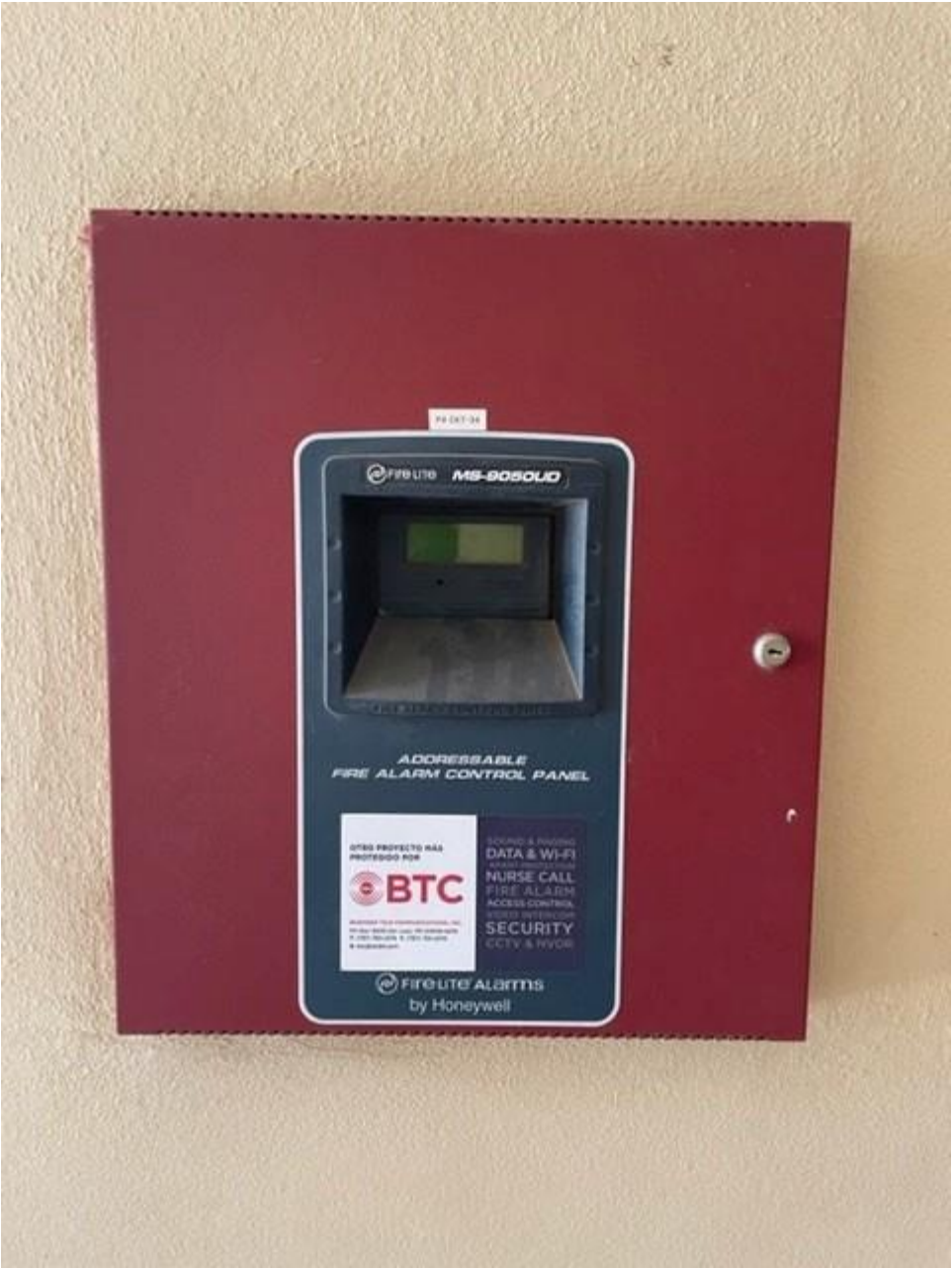
EXISTING FIRE ALARM CONTROL PANEL OF BUILDING 415: FOR REFERENCE ONLY
