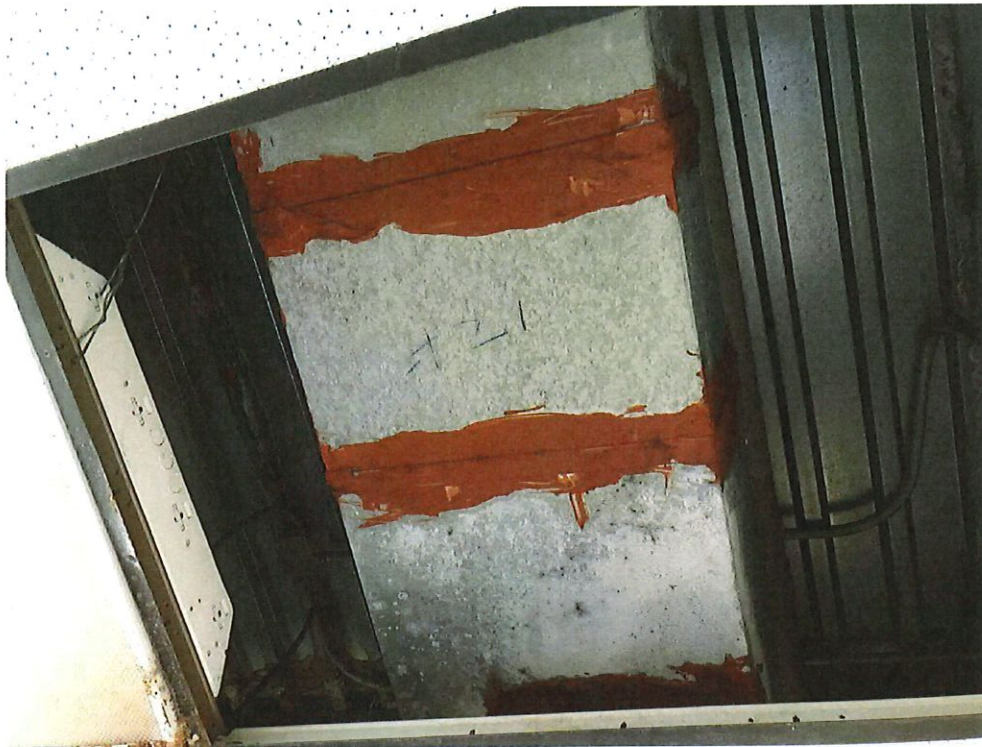
Photo Number 7 – Exam & Treatment Room Red Mastic Duct Air
