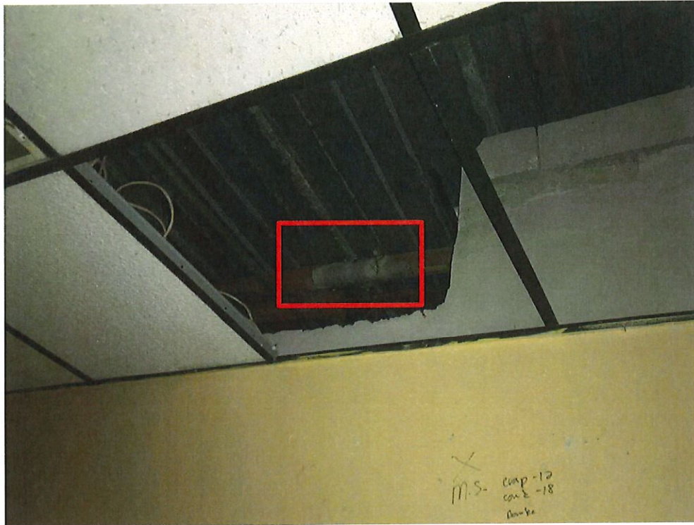
Photo Number 12- Hot Water Return Pipe Insulation
