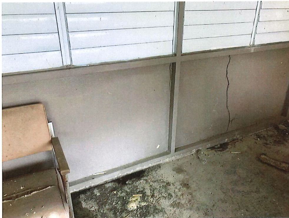
Photo Number 31 – Wall Interior "A" Loading Platform
