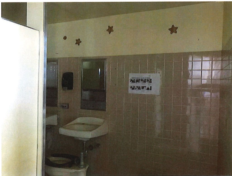
Photo Number 14 – Wall Interior Restrooms
