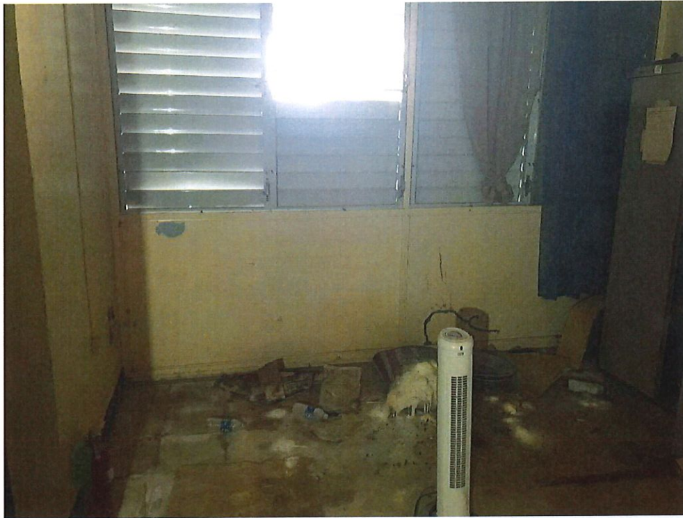
Photo Number 30 – Wall Interior "A" Soiled Linen
