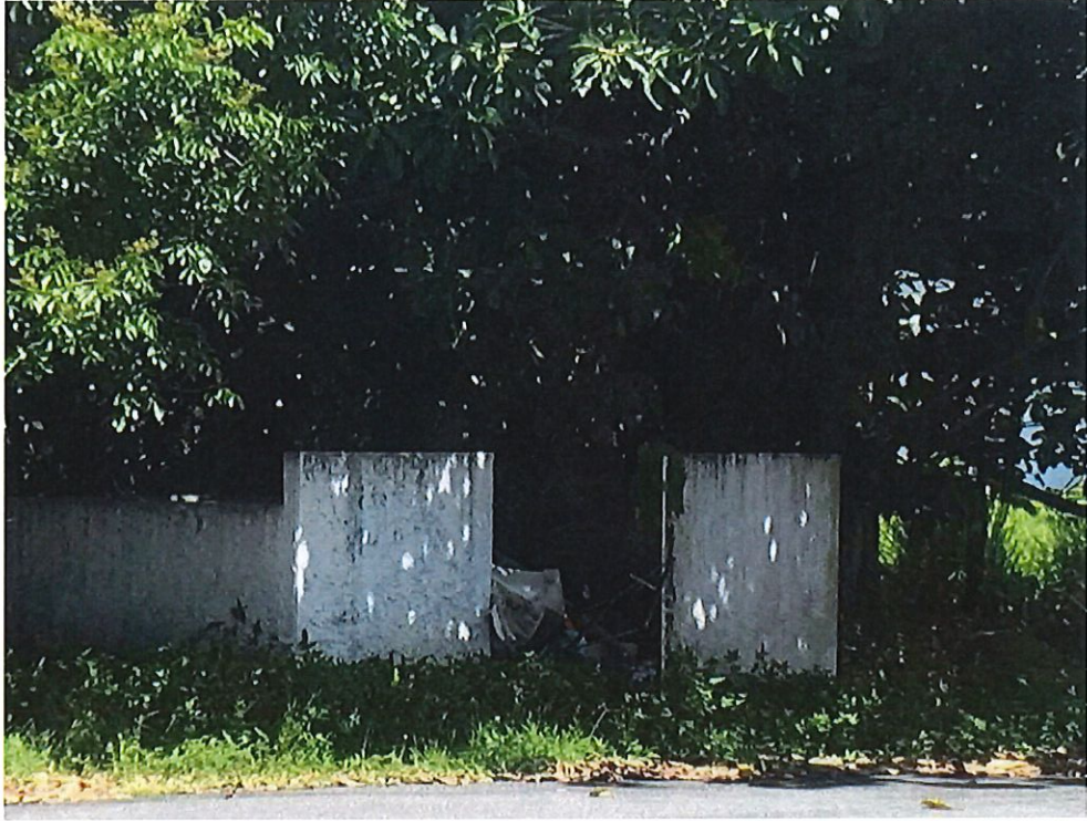
Photo Number 5 – Satellite Buildings (Garbage Station)
