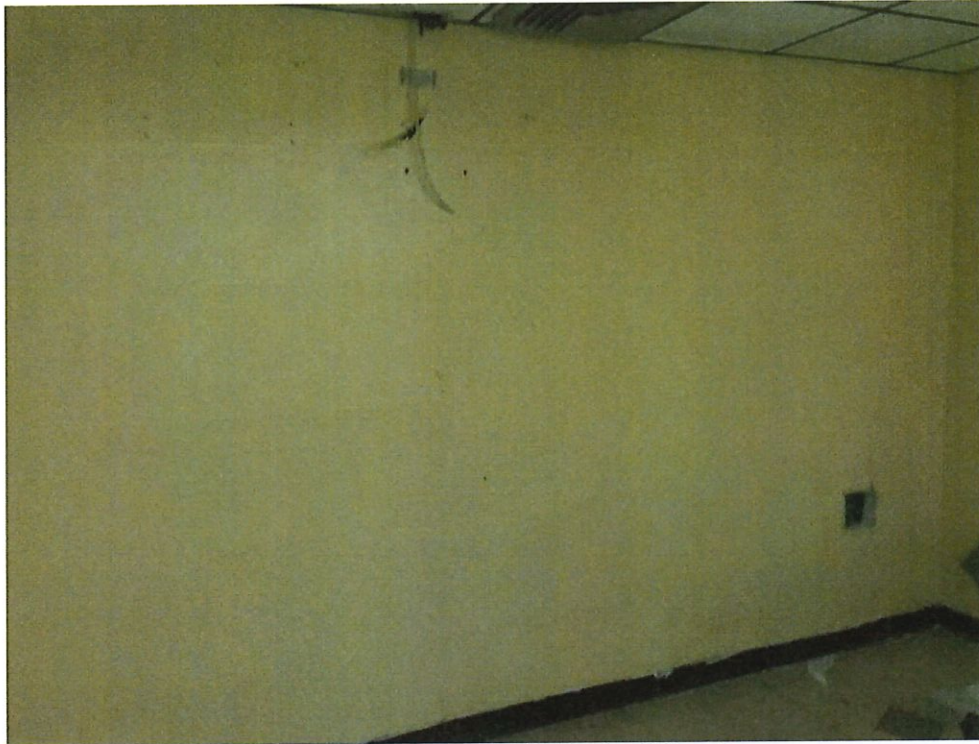
Photo Number 25 – Wall "B" Interior X-Ray Room
