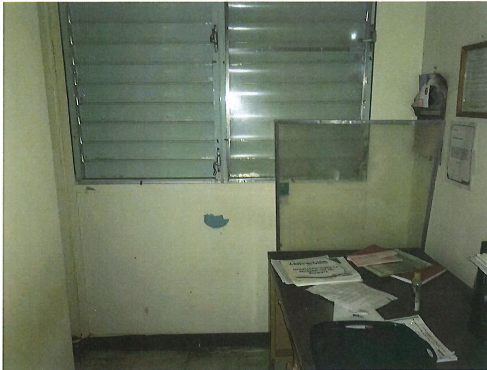
Photo Number 1 –Interior walls
