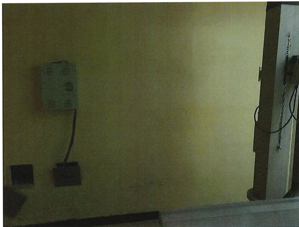
Photo Number 26 – Wall "D" Interior X-Ray Room
