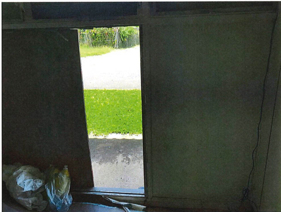
Photo Number 17 – Wall Interior "A" Exam & Treatment Room (71C)
