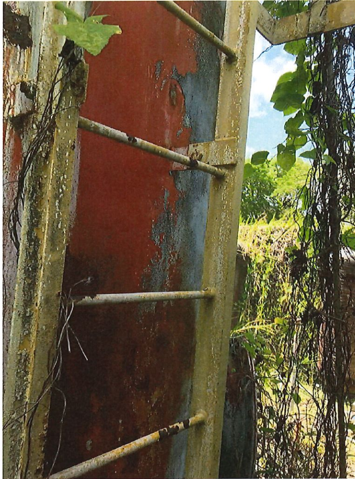
Photo Number 32 – Building Exterior Tank Stairs
