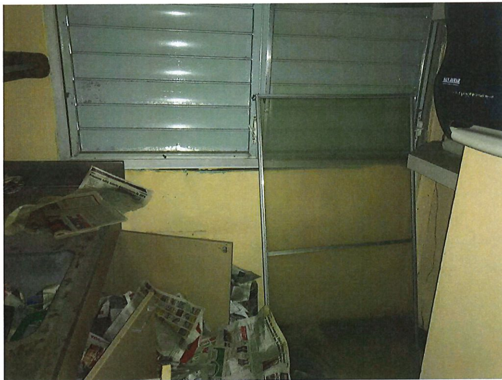
Photo Number 19 – Wall Interior “A” Clean Utility
