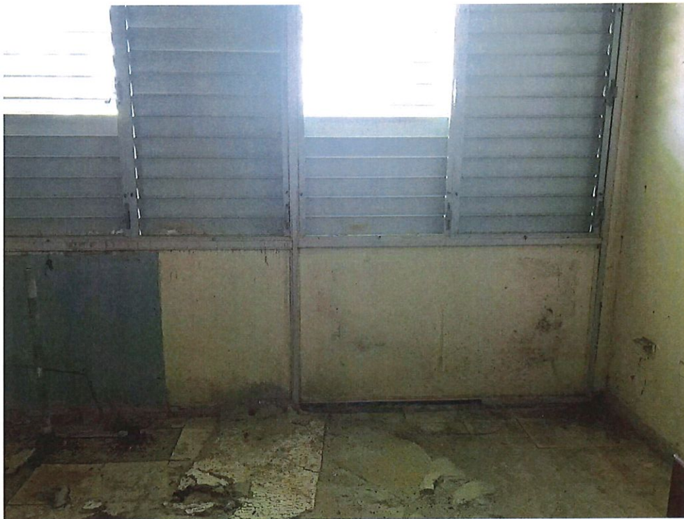
Photo Number 13 – Wall interior “D” Work Area
