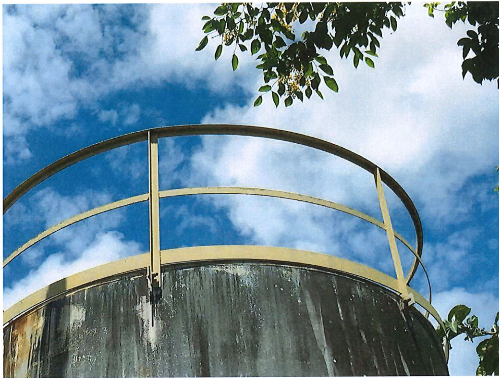
Photo Number 33 – Building Exterior Tank Handrail
