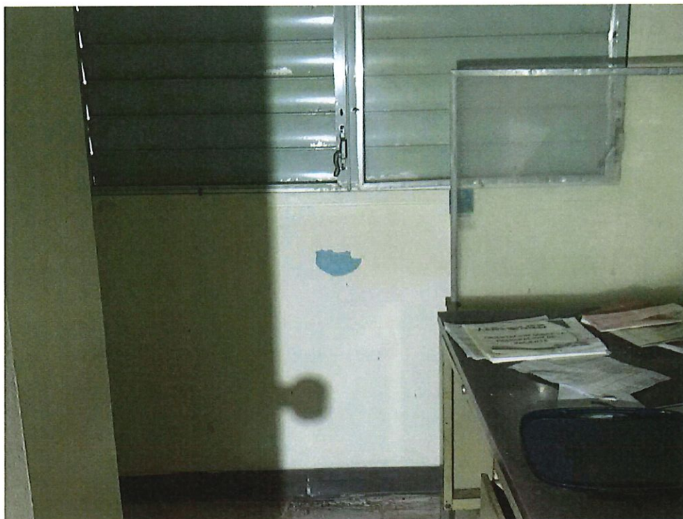
Photo Number 21 – Wall Interior “A” Soiled Utility
