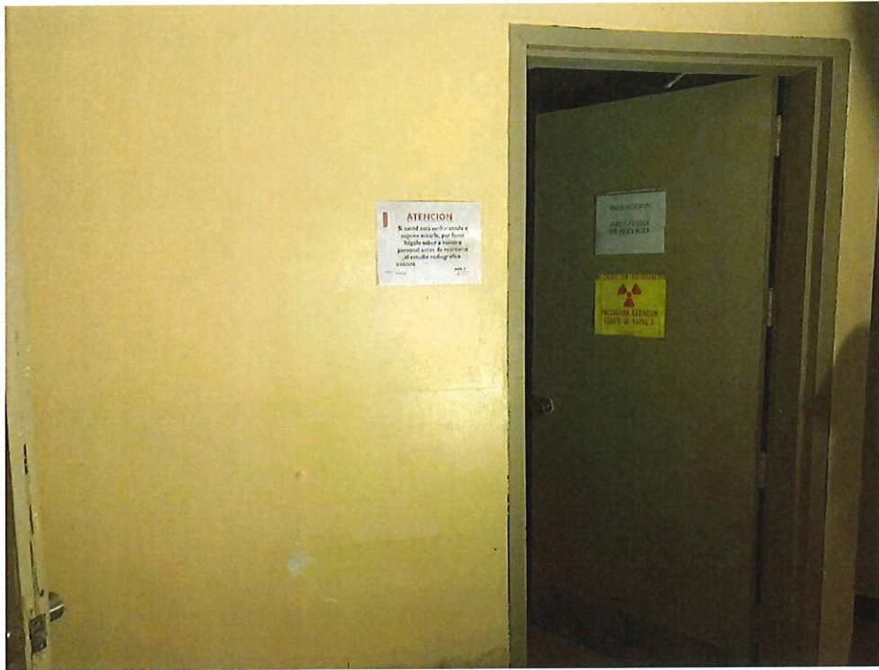
Photo Number 23 – Wall Interior “A” X-Ray Room
