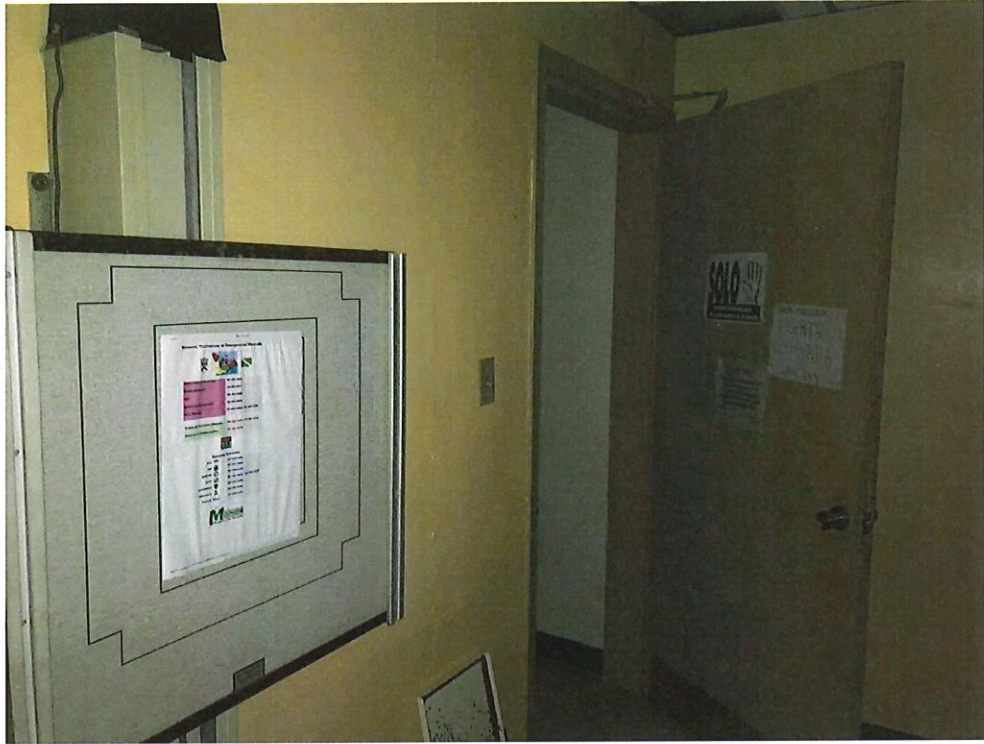
Photo Number 27 – Wall "C" Interior X-Ray Room
