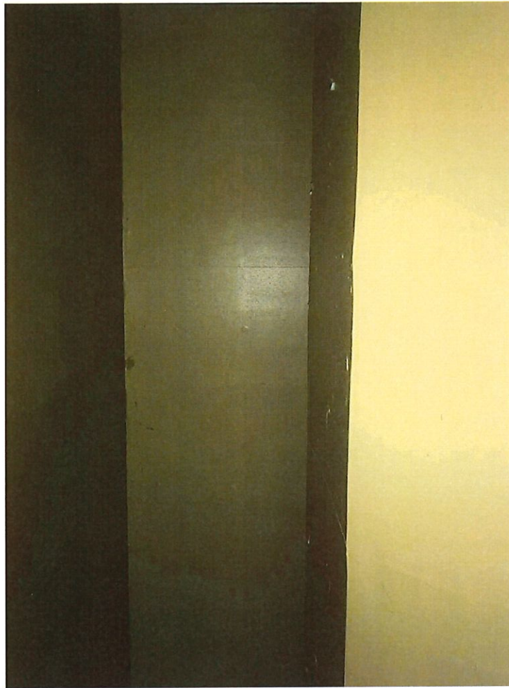
Photo Number 29 – Wall Interior Control X-Ray Room
