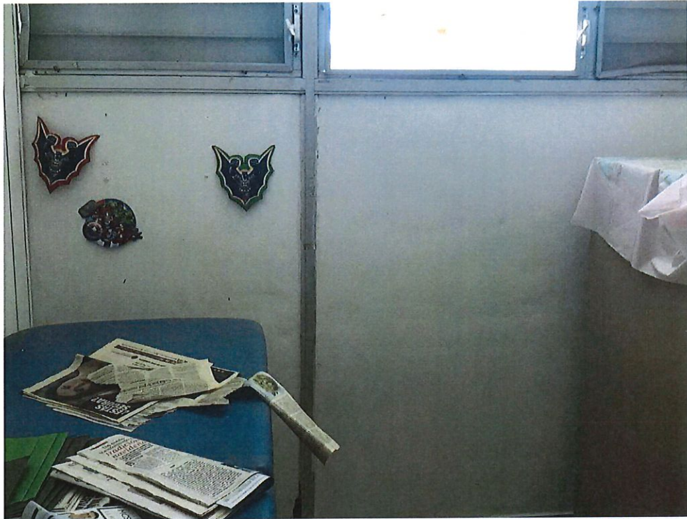
Photo Number 18 – Wall Interior “A” Exam & Treatment Room (70C)
