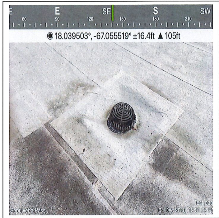
Lajas (CDT) roof temporary repair w/ insulation, roof drainage
