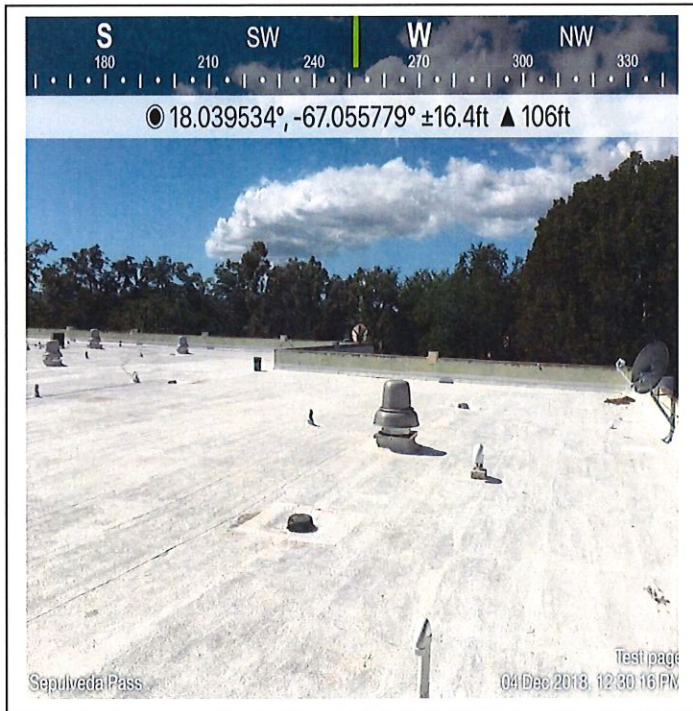
Lajas (CDT) roof temporary repair w/ insulation
