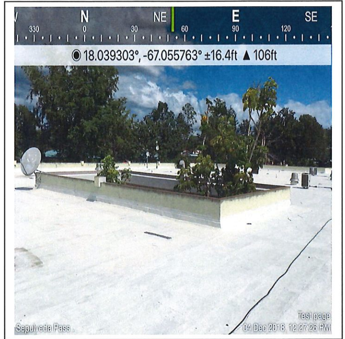
Lajas (CDT) roof temporary repair w/ insulation
