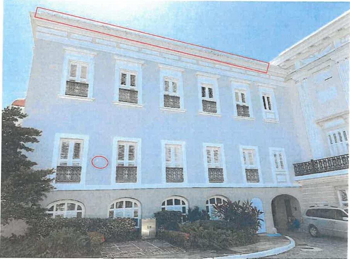
Pressure wash, repair concrete molding and fill cracks.
