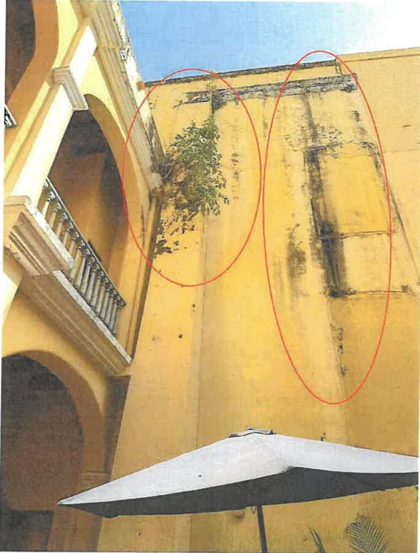
The interior patio has vegetative material to be removed and repaired.
