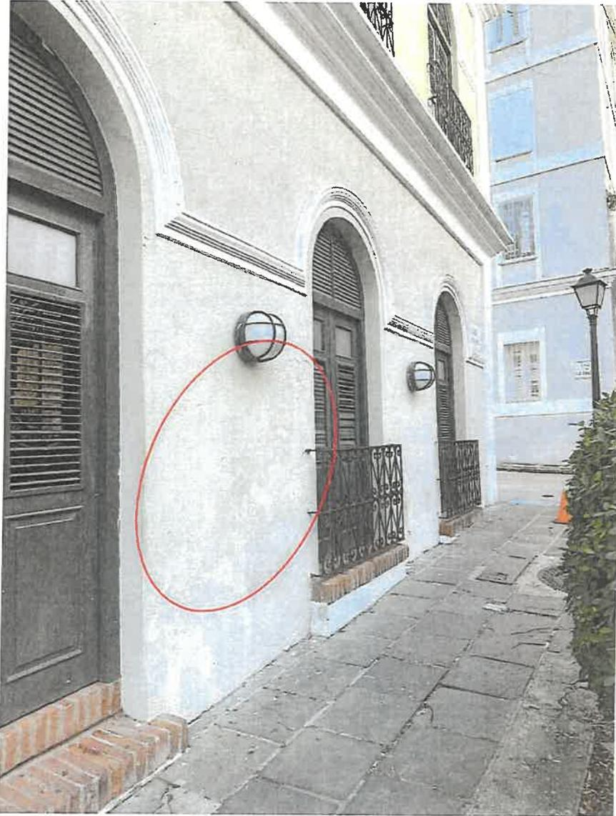
Seal cracks and pressure wash.
