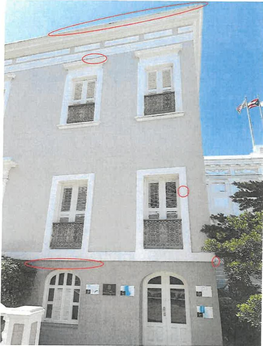
Seal all cracks, pressure wash, and repair the window concrete cornice.
