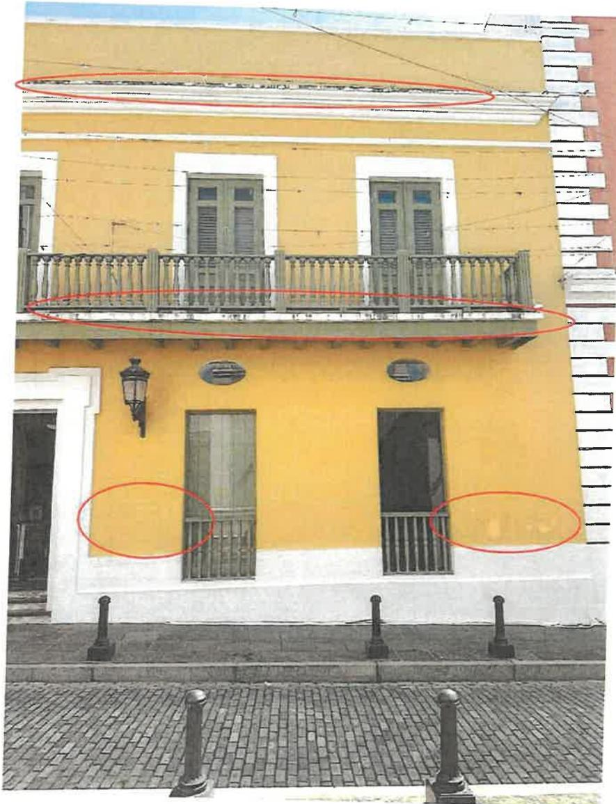
The building needs to be pressure washed and repair crack lines.
