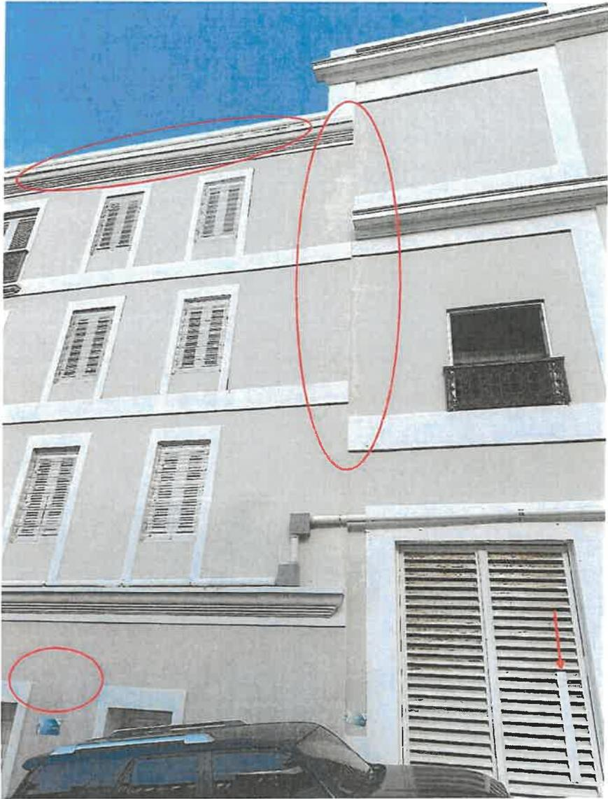
Seal cracks, pressure wash, repair concrete cornice and maintain parking lines.
