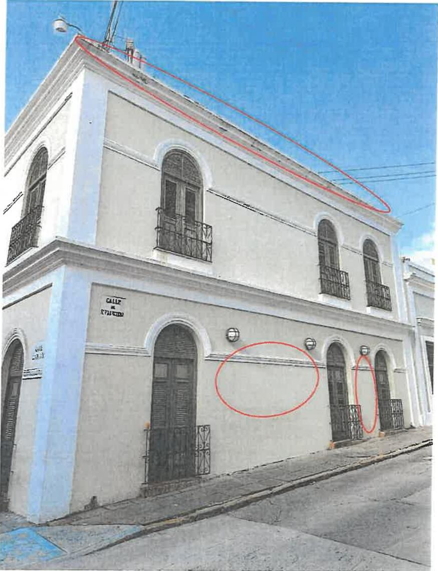
Repair all the concrete moldings with damage and seal all the cracks.
