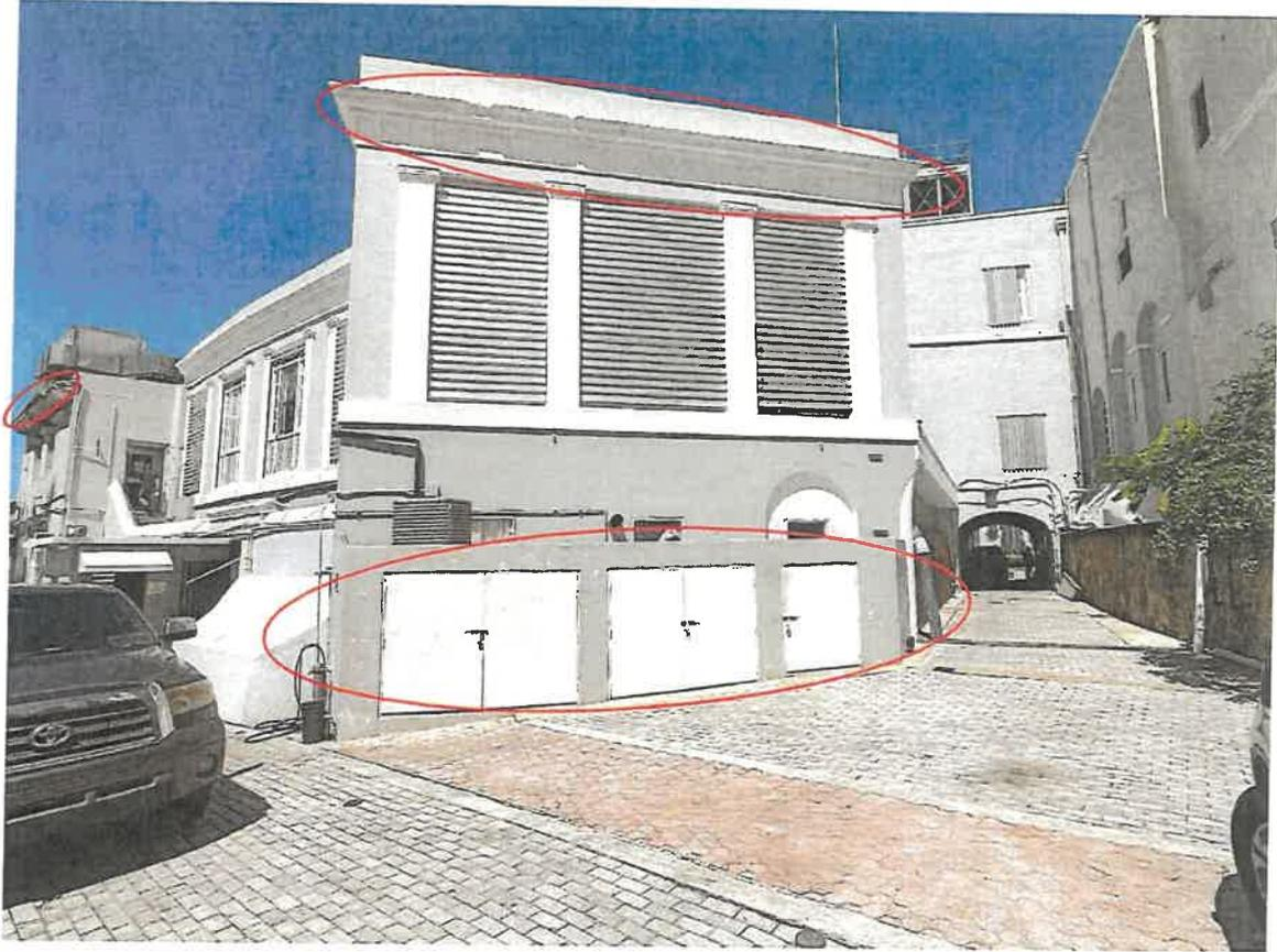
Repair concrete cornice, seal cracks, and remove vegetative material.
