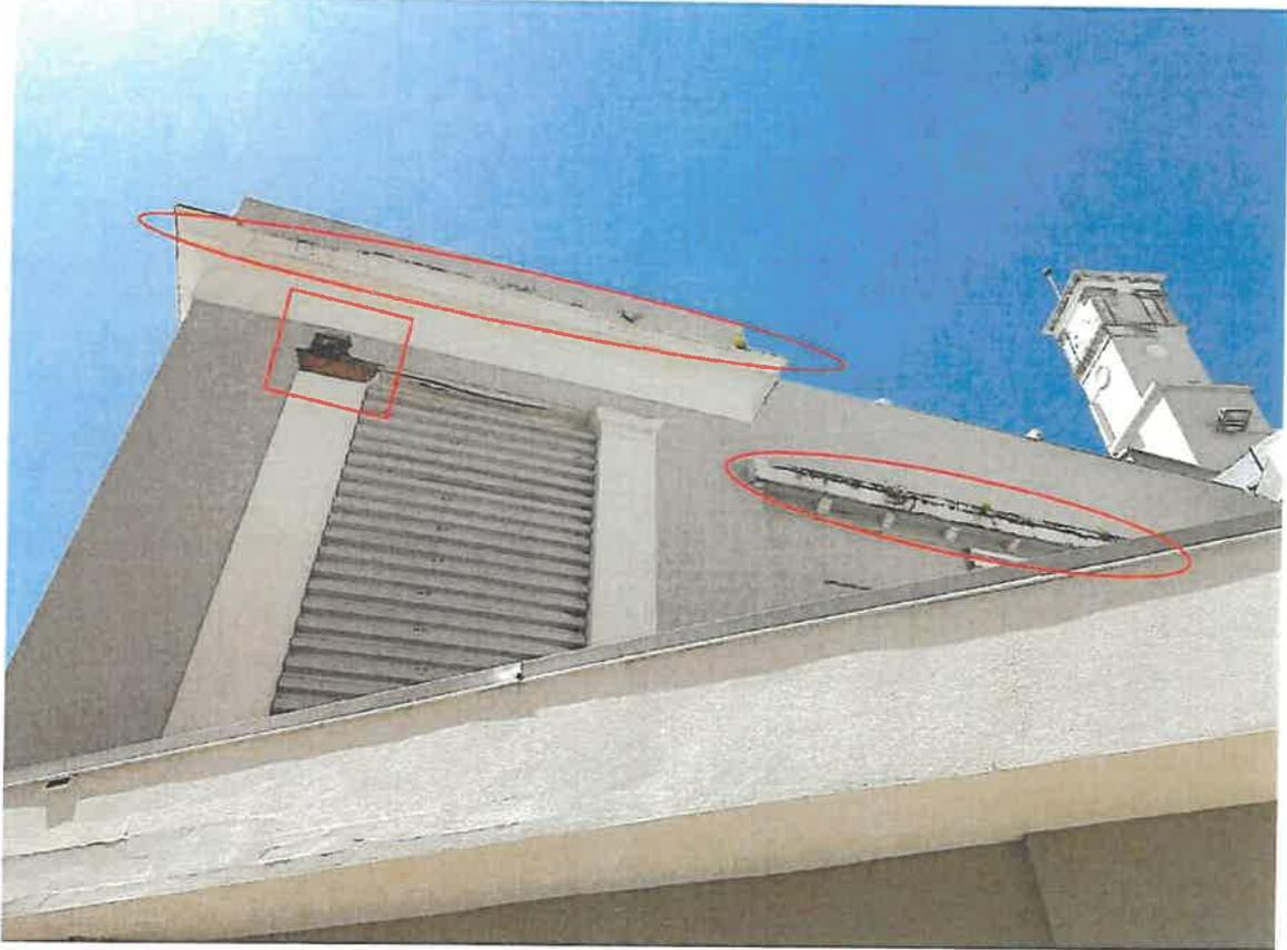
Repair concrete cornice, install the concrete cornice missing, and remove all vegetative material.
