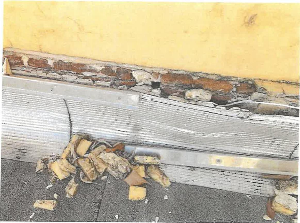
Bricks are exposed and the flashings need to be repaired, these is the wall adjacent to the weather tower.
