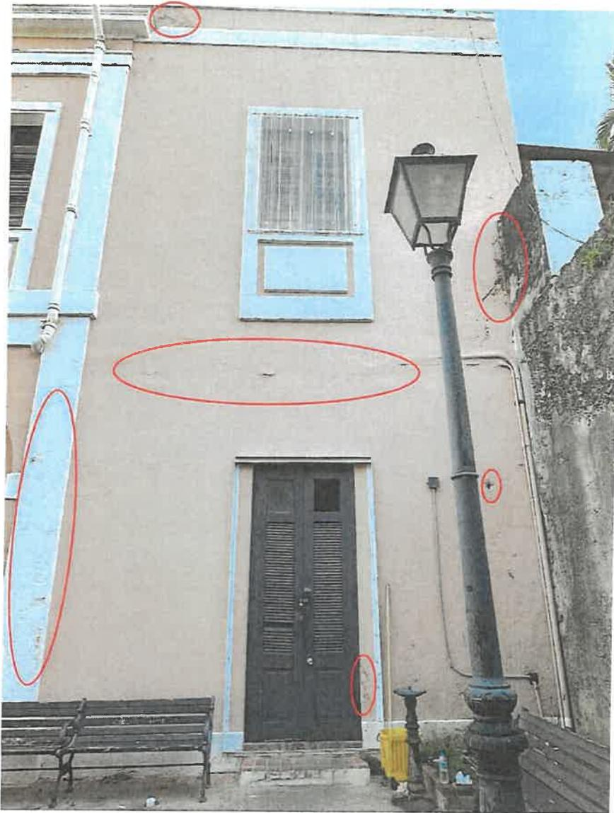
Repair walls, fill holes in concrete and repair concrete frames.
