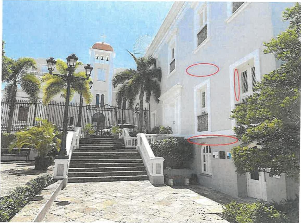
Fill cracks in walls and pressure wash.
