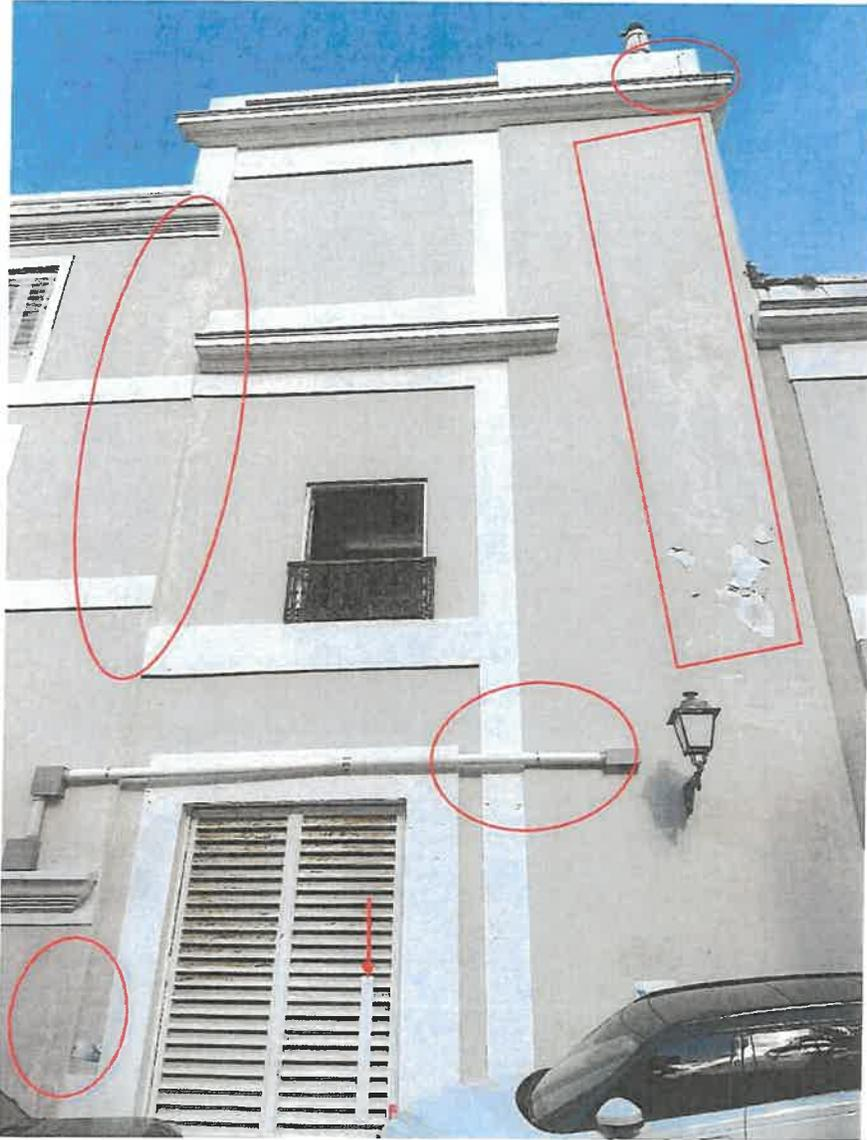
Pressure wash, maintain parking lines, repairs concrete cornice, and seal the crack lines.
