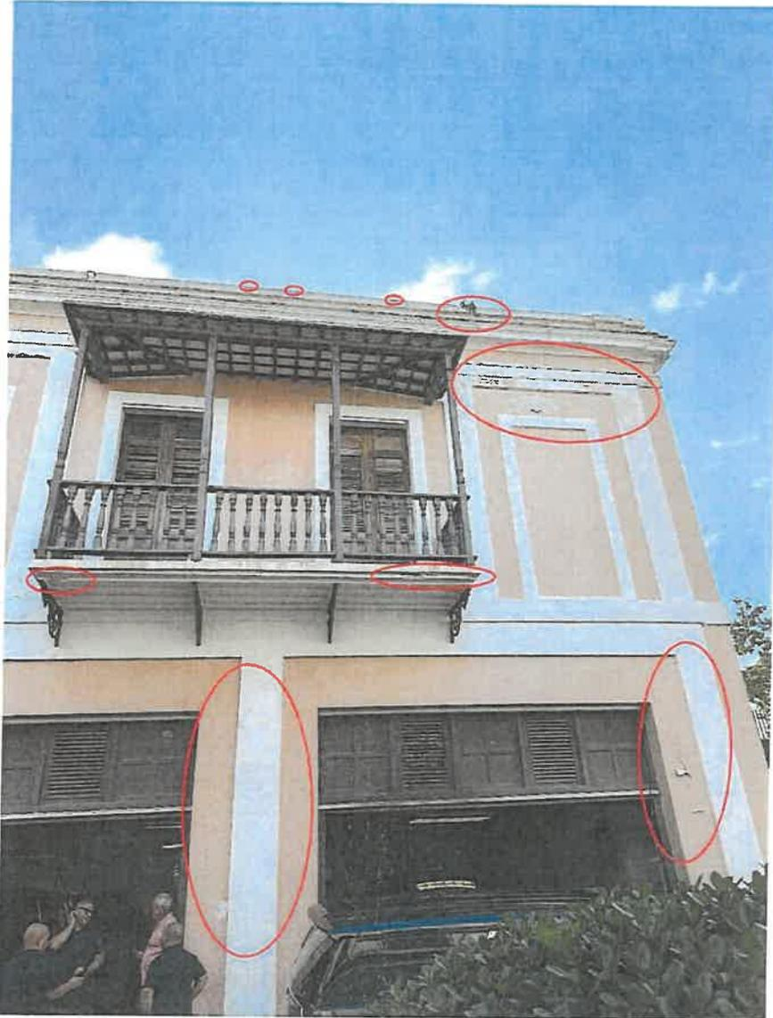
Seal cracks, repair balcony moldings and remove vegetative material.
