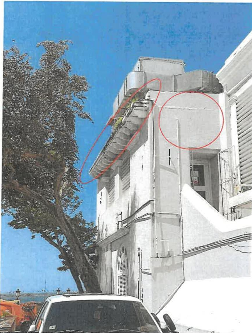
Pressure wash, seal cracks, and remove vegetative material in the concrete cornice.
