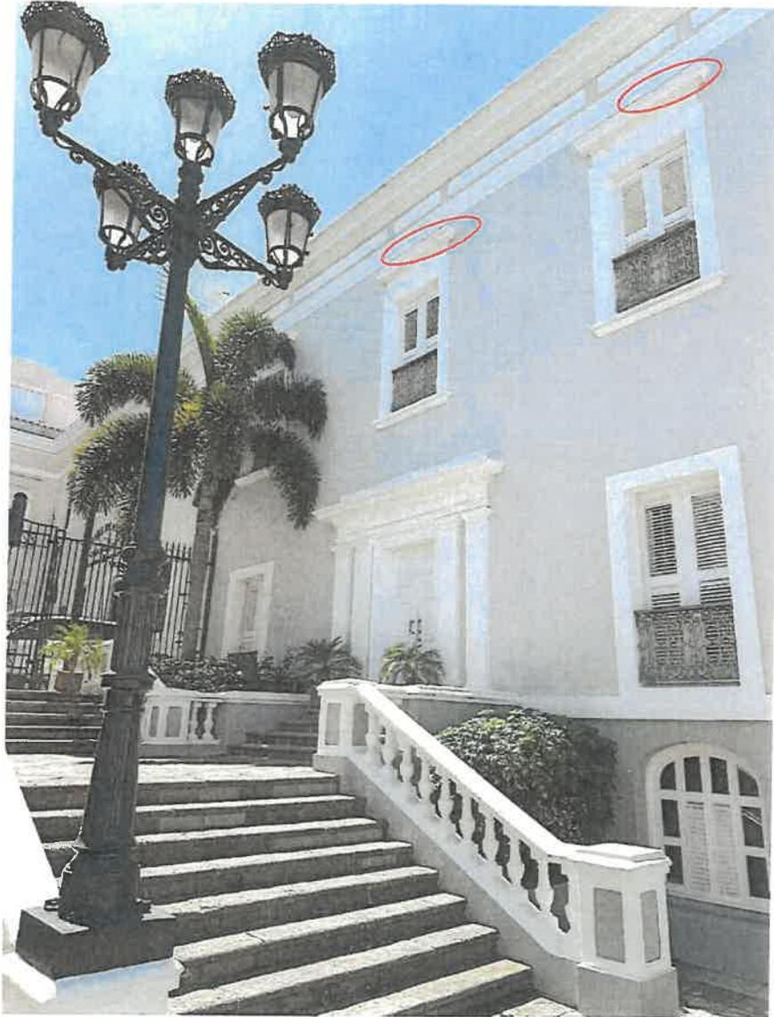
Repair windows concrete cornice, pressure wash, and fill cracks.
