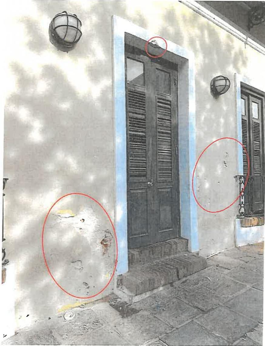
Repair concrete frame at doors, repair concrete plaster and fill cracks.
