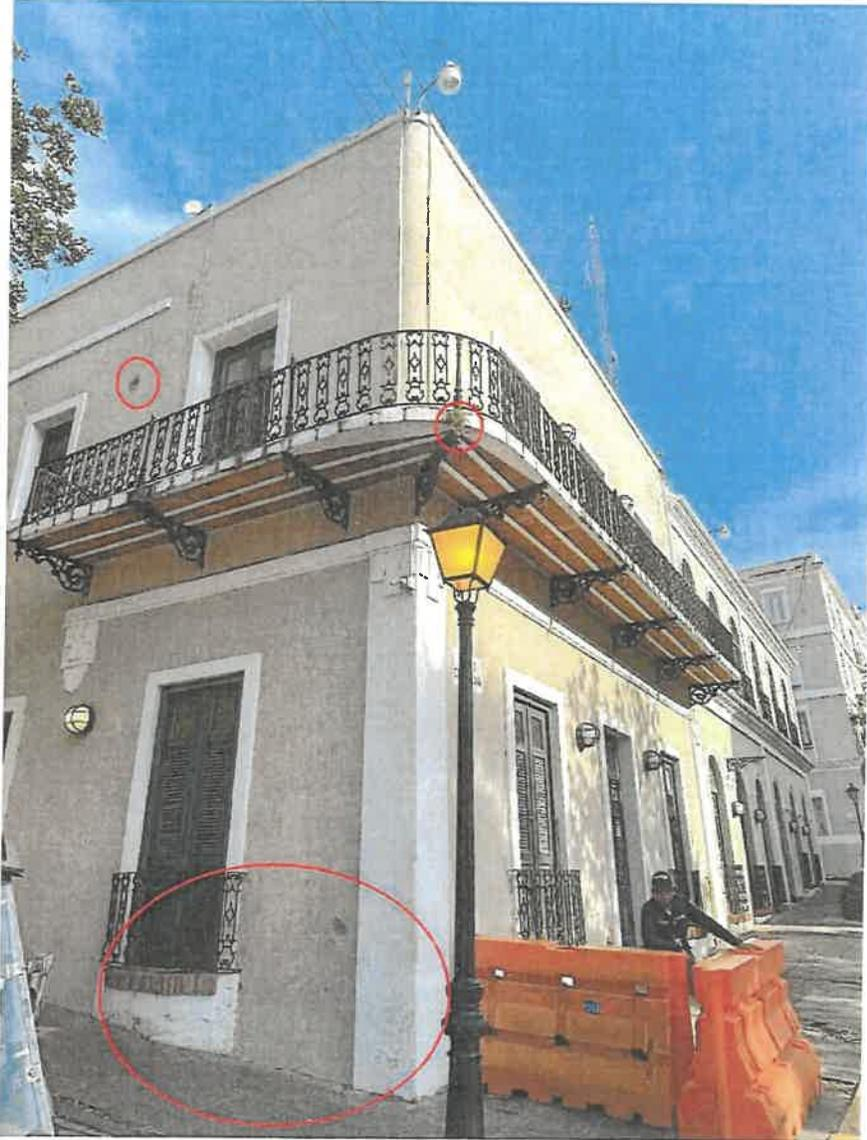
Remove all vegetative material and fill cracks.
