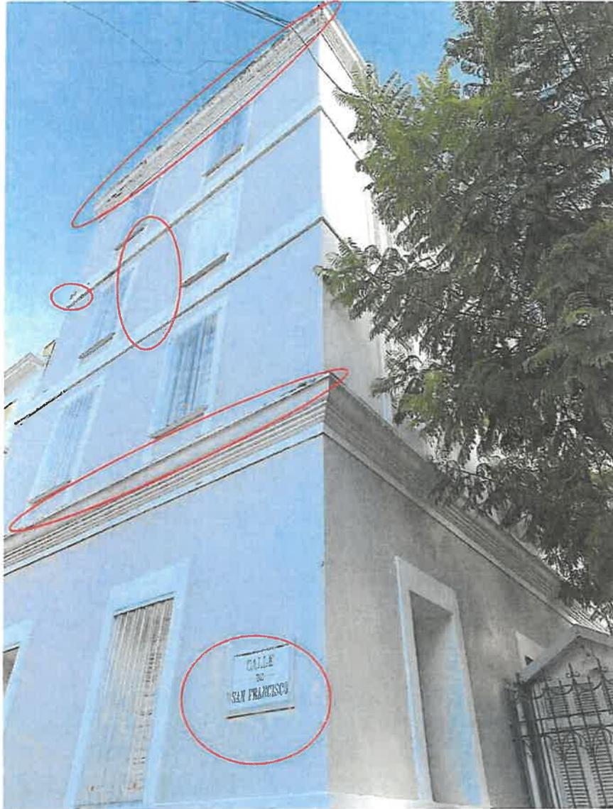
Seal all crack lines, repair concrete cornice, and pressure wash.
