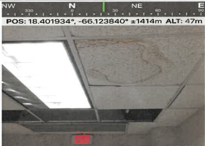
Basement – Acoustic Ceiling Tiles
