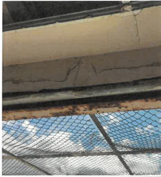
3 rd Floor Roof Covered Area - Soffit Gypsum Board
