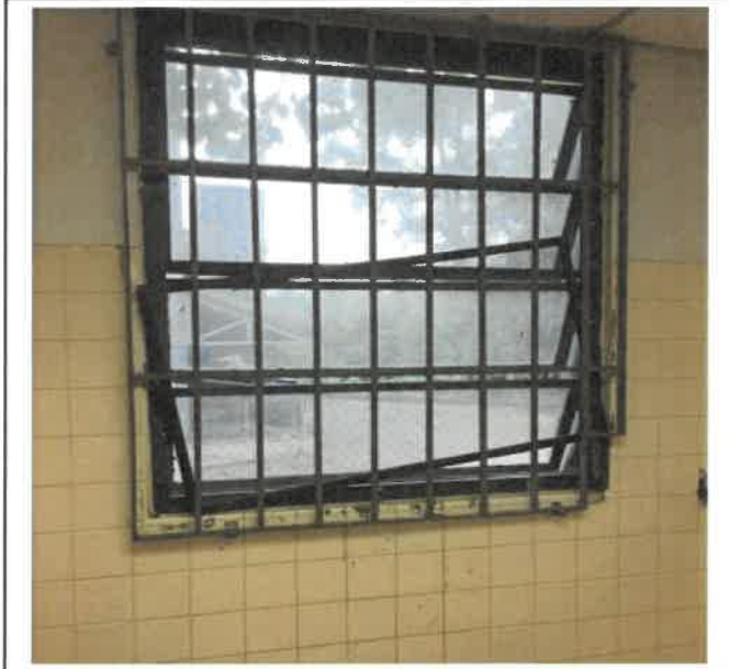
Basement Morgue – Jalousie Aluminum Window
