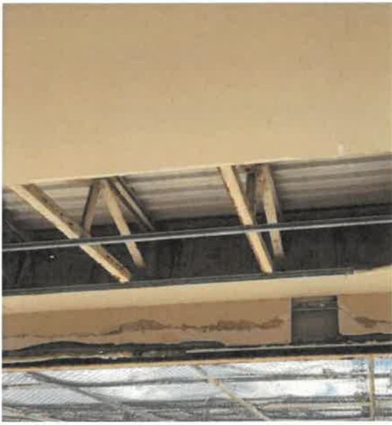
3 rd Floor Roof Covered Area - Ceiling & Soffit Gypsum Board
