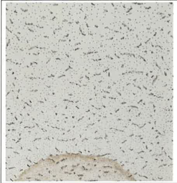
Ground Floor – Acoustic Ceiling Tiles
