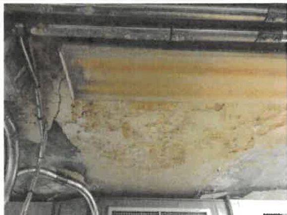
Photo 34 – UPS Room, damaged concrete ceiling plaster (cracked and detached)
