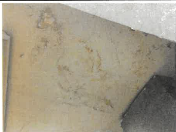
Photo 33 – UPS Room, damaged concrete ceiling plaster (cracked and detached)
