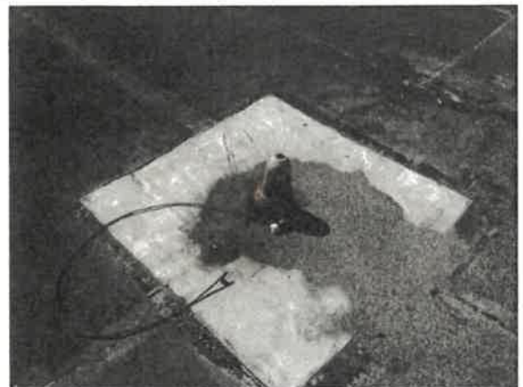
Photo 50 – Minisplit A/C unit was knocked down and disconnected (was re-connected as an immediate, temporary measure)
