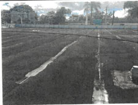
Photo 41 – Damaged roof waterproof system (bitumen rolls), scrapped, detached, and bubbled
