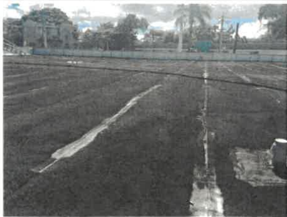
Photo 41 – Damaged roof waterproof system (bitumen rolls), scrapped, detached, and bubbled
