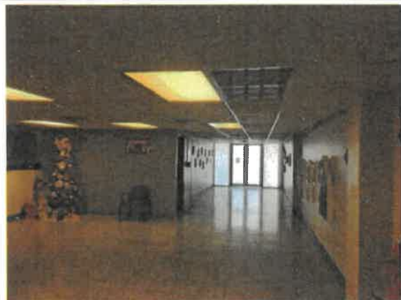
Photo 9 – Lobby / Pharmacy area, damaged acoustic tiles (2 FT wide by 4 FT height)
