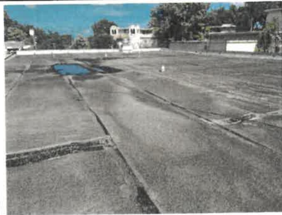
Photo 42 – Damaged roof waterproof system (bitumen rolls), scrapped, detached, and bubbled
