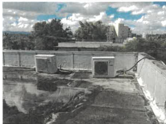
Photo 46 – Damaged 10 FT roof parapet wall section, bended and broken
