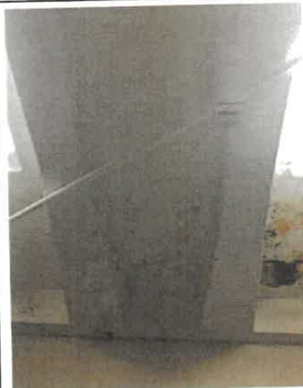
Photo 14 – Pharmacy Area / Materials Storage, concrete ceiling paint, 28 FT long x 11 FT wide, peeled paint due to water intrusion from 2nd floor
