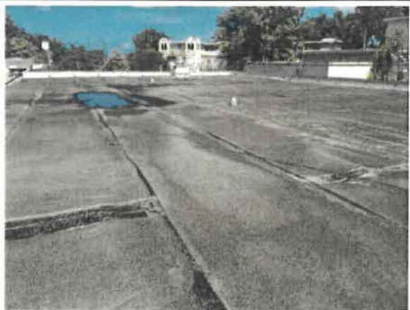
Photo 42 – Damaged roof waterproof system (bitumen rolls), scrapped, detached, and bubbled
