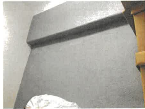
Photo 26 – OCASET File Room, damaged concrete wall paint, 14.75 FT long x 10 FT wide, bubbled paint due to water intrusion
