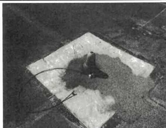
Photo 50 – Minisplit A/C unit was knocked down and disconnected (was re-connected as an immediate, temporary measure)
