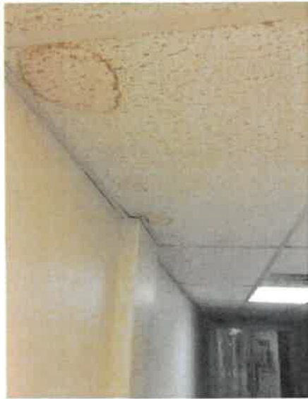
Photo 25 – Hallway, OCASET, damaged acoustic tiles (2 FT wide by 4 FT height)
