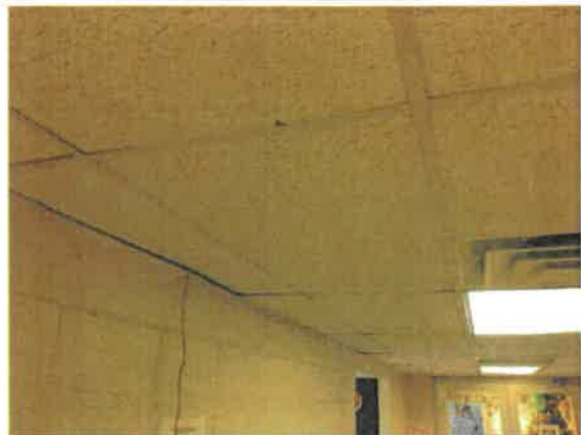
Photo 10 – Lobby / Pharmacy area, damaged acoustic tiles (2 FT wide by 4 FT height)
