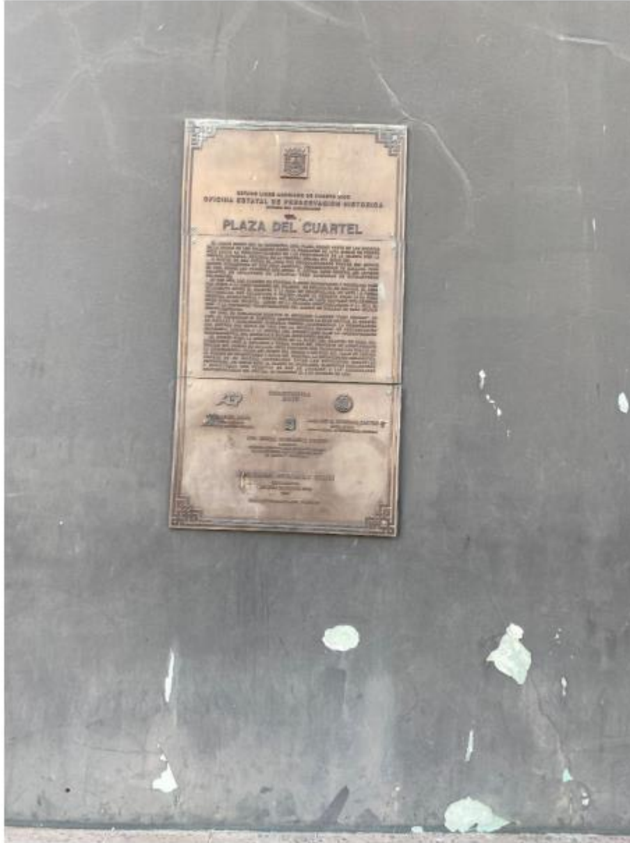
Photo 3 Prior to commencing work, the contractor shall remove all the plates, deliver it to the owner for storage and coordinate installation upon completion of the work.
