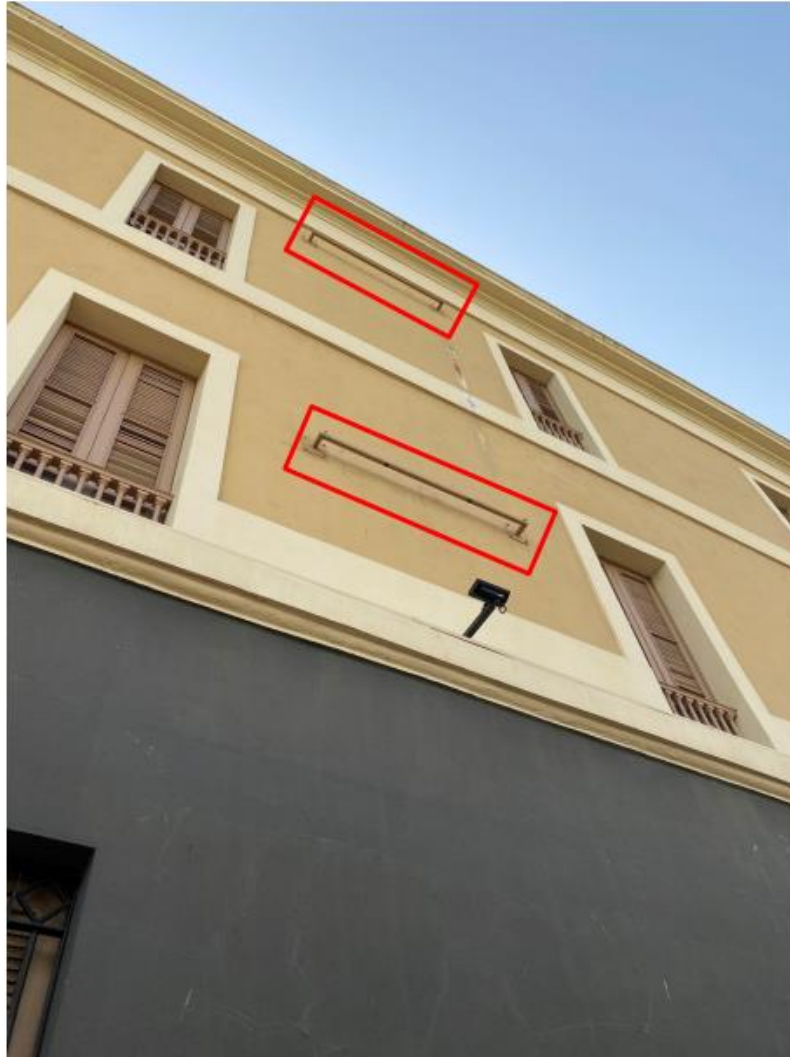
Photo 1 Contractor shall remove and replace with new stainless steel frame, according to the construction drawings.
