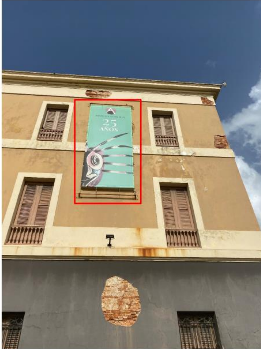
Photo 2 Contractor shall remove and replace with new stainless steel frame, according to the construction drawings. Banner will be removed and delivered to owner.
