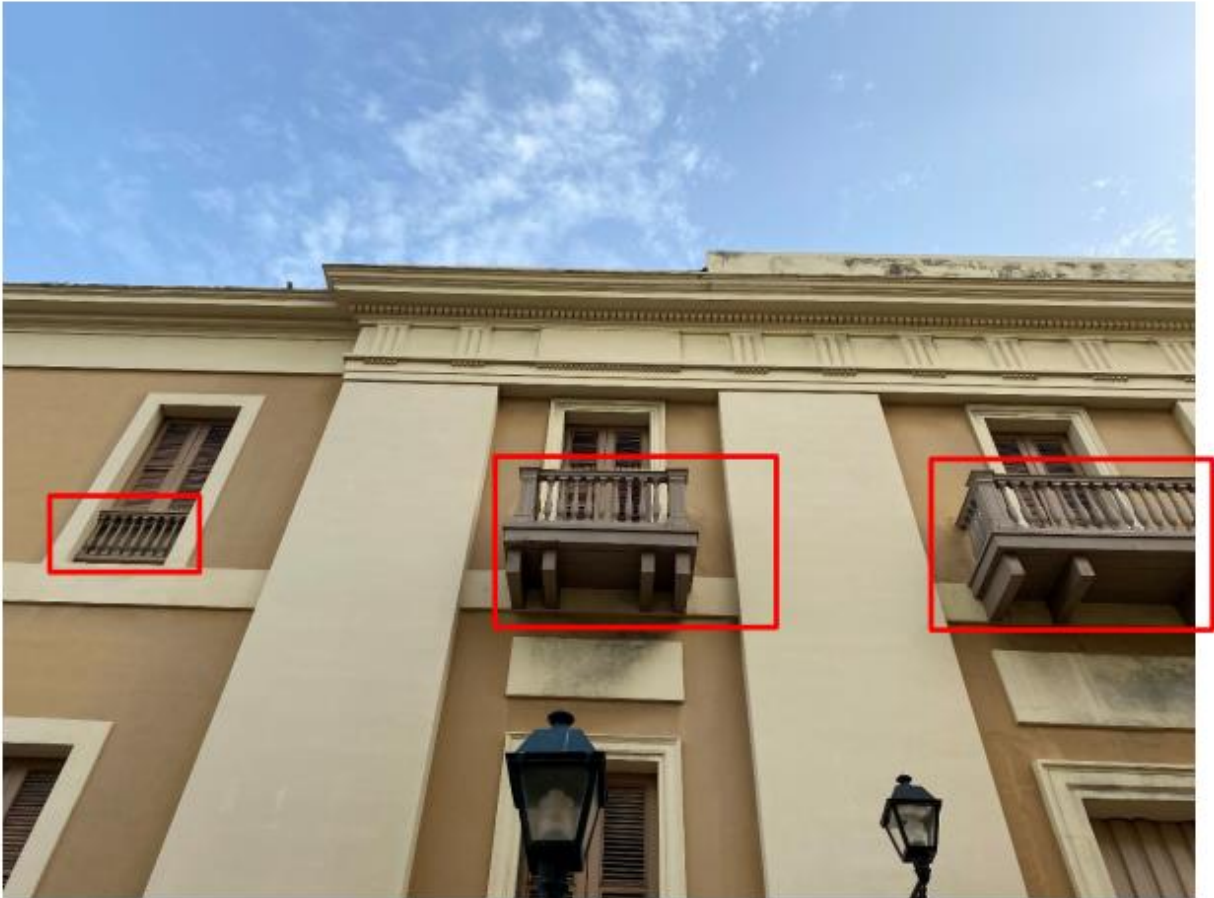
Photo 4 The contractor should consider painting and repairing, as necessary, wooden balconies and balusters
