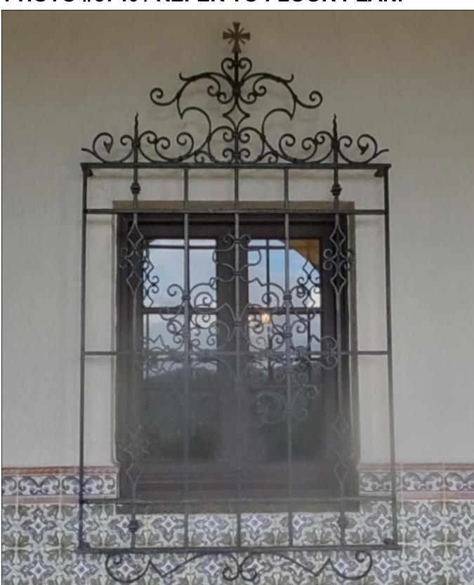
G.C. SHALL REFINISH WINDOW GRILLE ELEMENTS. WINDOW GRILLE REFINISHING SHALL BE WORKED ON IN PLACE, THERE IS NO NEED TO REMOVE. G.C. SHALL NOT BREAK OR DETACH WALL PLASTERING. SEE FINISH NOTES FOR ADDITIONAL INFORMATION. | THIS REPAIR BELONGS TO ALTERNATE B.
