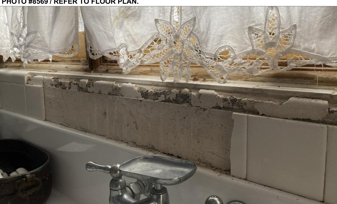
G.C. SHALL REMOVE ALL SHOWN DAMAGED PORTION OF KITCHEN WALL TILES AND REPLACE WITH NEW. G.C. SHALL REQUEST EXISTING TILES STORED BY OWNER AND USED THOSE TO THIS REPAIR. IN THE CASE THAT MORE TILES ARE NEEDED TO COVERED ALL THE DAMAGED AREA, NEW TILES SHALL BE BY AMERICAN OLEAN MATCHING EXISTING. | CERAMIC TILE GROUT SHALL ALSO MATCH EXISTING. | THIS REPAIR BELONGS TO ALTERNATE A.
