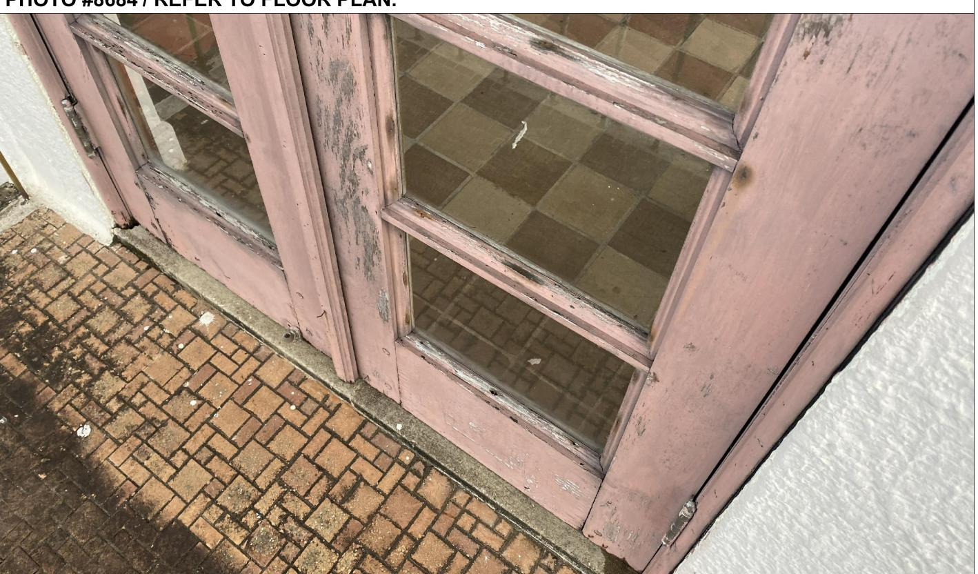
G.C. SHALL REMOVE AND REPLACE EXISTING DOOR AND FRAME ON WOOD DOOR MKD "38" FOR NEW. | EXISTING DOOR HARDWARE, SHALL BE REMOVED, REFINISHED AND REINSTALLED ON NEW DOOR. | REFER TO DOOR NOTES AND DETAILS FOR ADDITIONAL INFORMATION.
