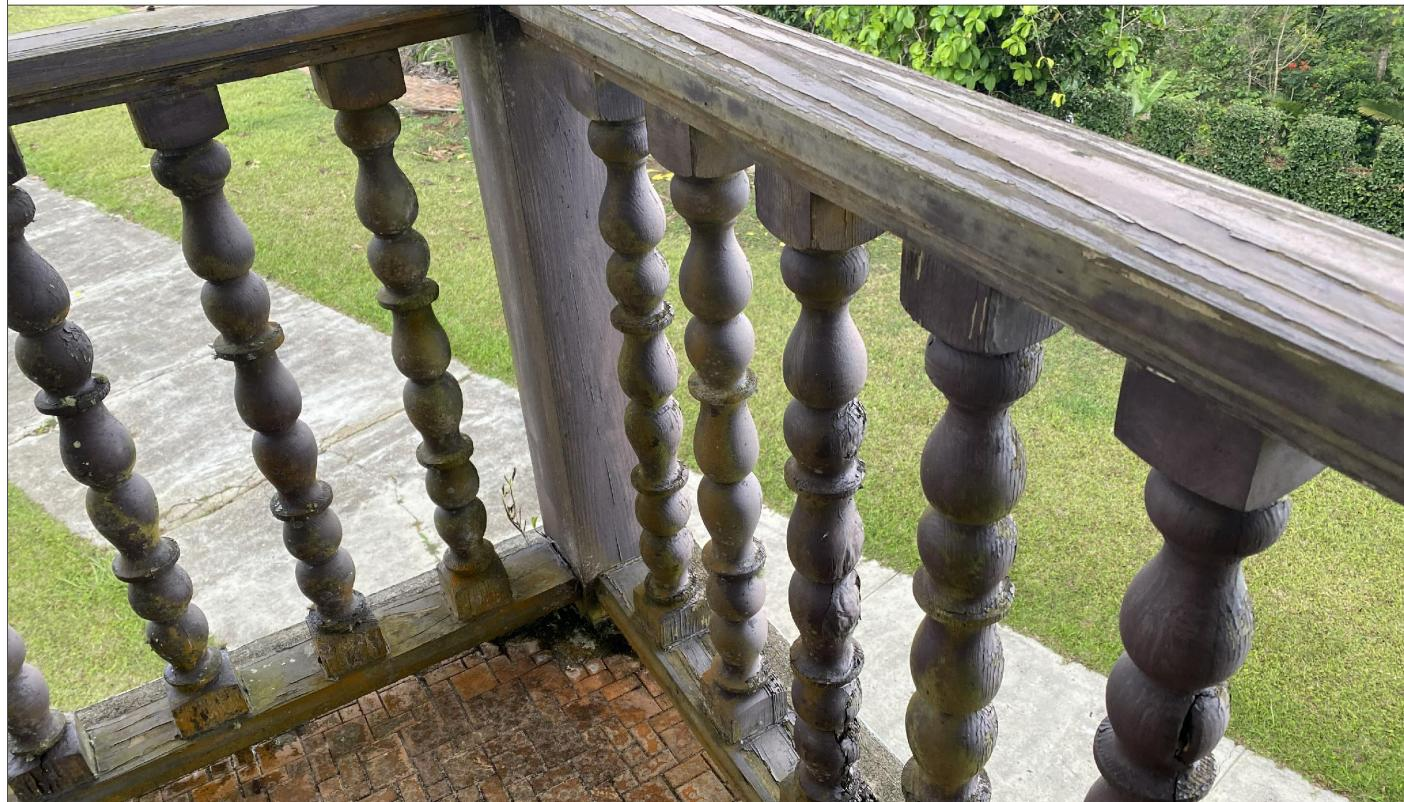
G.C. SHALL REFINISH BALUSTRADE. | BEFORE PROCEEDING, G.C. SHALL TAKE GENERAL AND CLOSE UP IMAGES OF BALUSTRADE'S CURRENT CONDITIONS FOR A/E REVIEW. | ENTIRE RAILING AND BALUSTERS SHALL BE THOROUGHLY SCRAPPED FROM EXISTING PAINT BEFORE REPAINTING, SEE SPECS. | FOR WOOD REPAIR INSTRUCTIONS SEE SPECS. | THIS REPAIR BELONGS TO ALTERNATE B.
