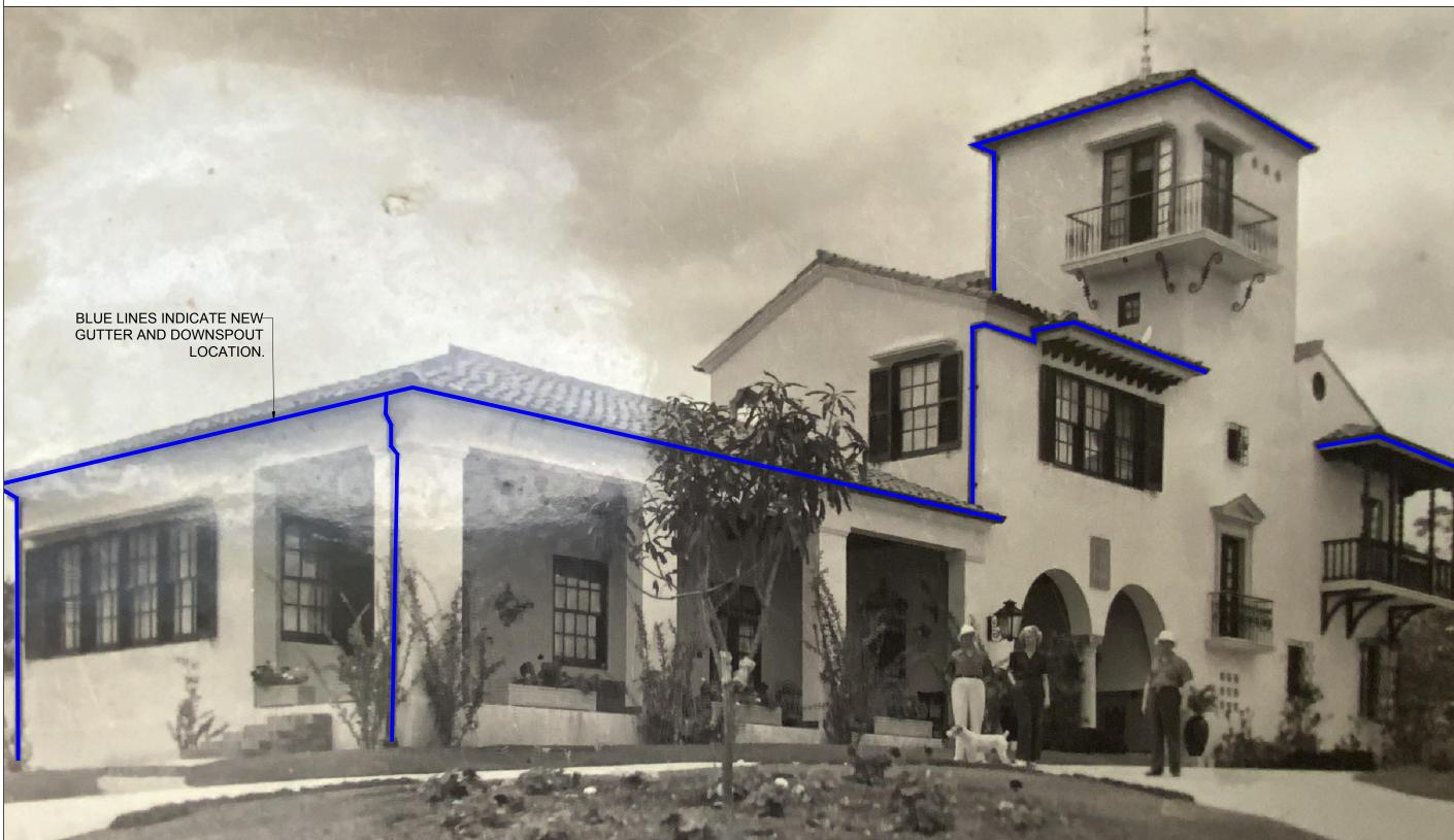
G.C. SHALL INSTALL NEW COPPER GUTTER AND DOWNSPOUTS AND CONNECT THEM TO THE EXISTING SYSTEM THAT LEADS TO THE EXIST. CISTERN. | REFER TO ELEVATIONS AND ROOF IN ORDER TO PROPERLY LOCATE GUTTERS AND DOWNSPOUTS. | FINAL LOCATION OF GUTTERS AND DOWNSPOUTS SHALL BE DISCUSSED WITH OWNER AND ARCHITECT BEFORE PROCEEDING. | WHEN INSTALLATION OCCURS, G.C. NEEDS TO BE CAREFUL IN PROTECTING ROOF TILES. IF SOME MAY BREAK, G.C. SHALL SUBSTITUTE ACCORDINGLY. | SEE ALSO SHEETS A-04 & A-05.
