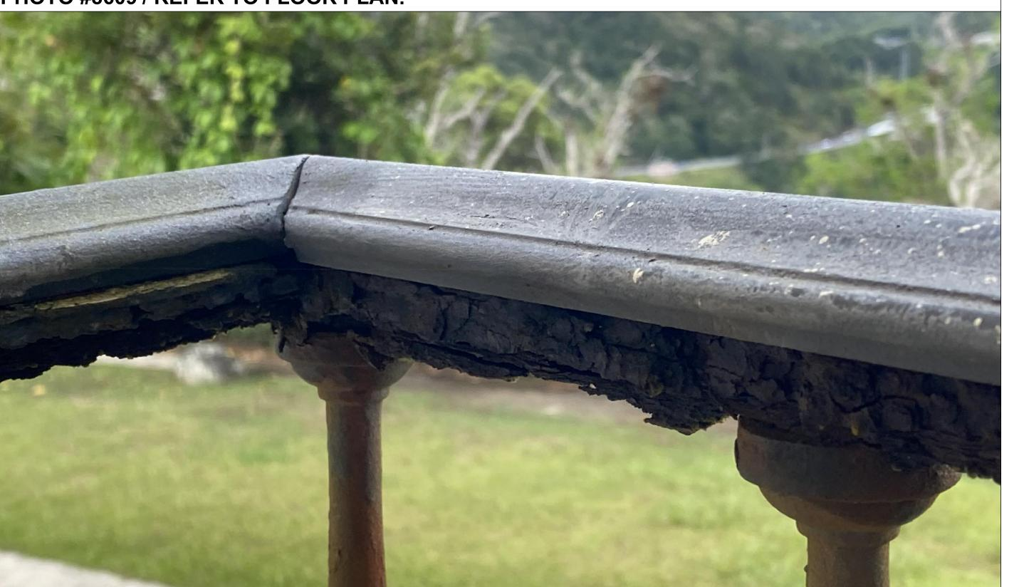
G.C. SHALL REMOVE ENTIRE CORRODED TOP RAIL AND REPLACE WITH NEW MATCHING EXISTING SHAPE, QUALITY, MATERIAL, FINISH, SIZE AND DIMENSION. | G.C. SHALL MAKE SURE METAL BALUSTERS ARE IN GOOD CONDITIONS, IF ANY BALUSTER IS DAMAGED AND/OR CORRODED, IT SHALL BE REPLACED BY NEW MATCHING EXISTING DESIGN. | SEE FINISH NOTES FOR ADDITIONAL INFORMATION.
