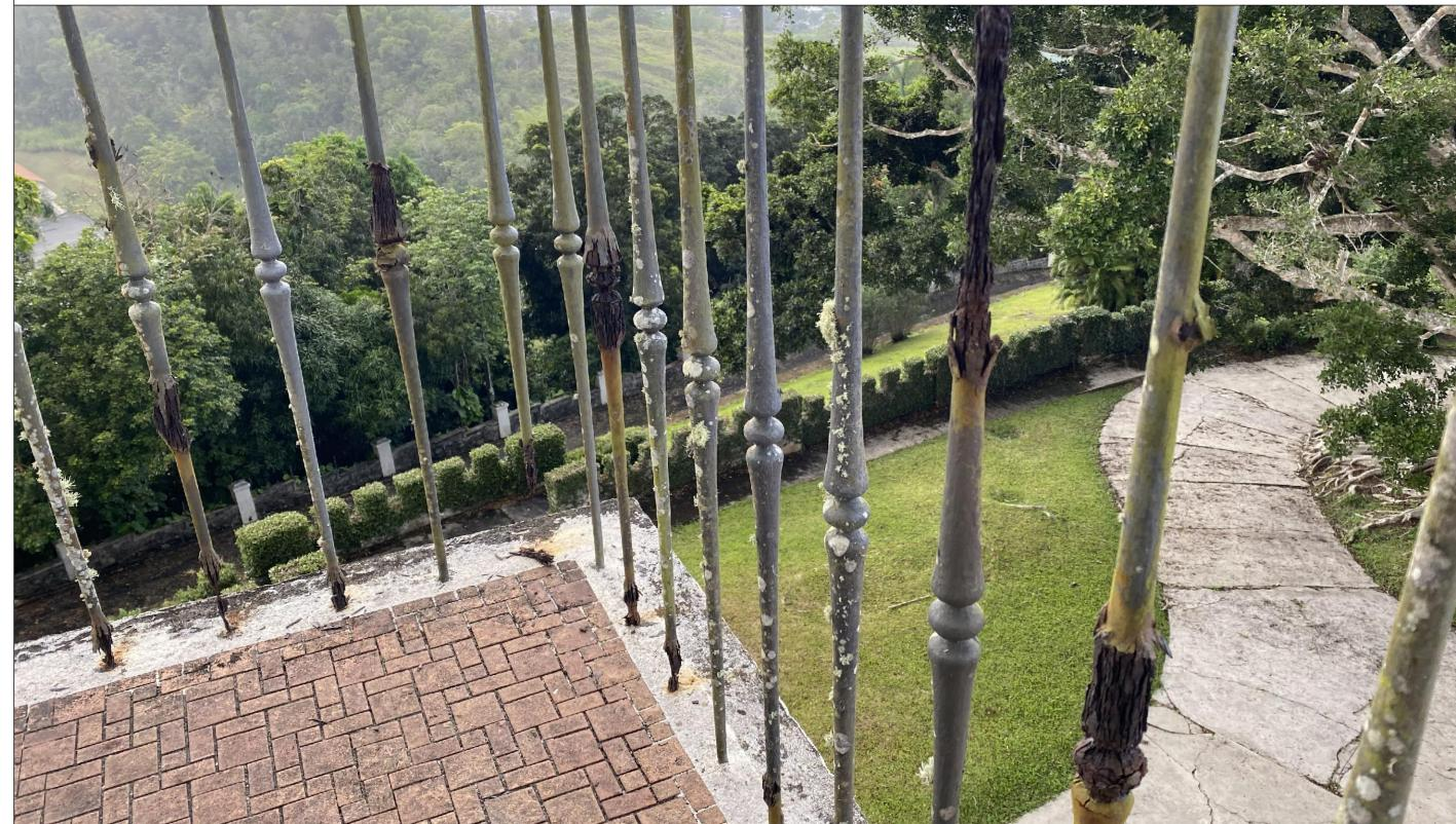
G.C. SHALL REMOVE AND REPLACE EXISTING METAL RAILING & BALUSTERS FOR NEW. | NEW RAILING & BALUSTERS DESIGN SHALL BE EQUAL IN MATERIAL, QUALITY, SHAPE, SIZE AND DIMENSION TO THE VERTICAL ELEMENTS LOCATED AT THE MAIN STAIR RAILING. | G.C. SHALL PROVIDE SHOP DRAWING BEFORE MANUFACTURING. | LEAD-BASED PAINT FOUND ON METAL RAILING ACCORDING TO LBP REPORT. G.C. SHALL BE RESPONSIBLE FOR FOLLOWING PROPER LEAD ABATEMENT PROCEEDURE.
