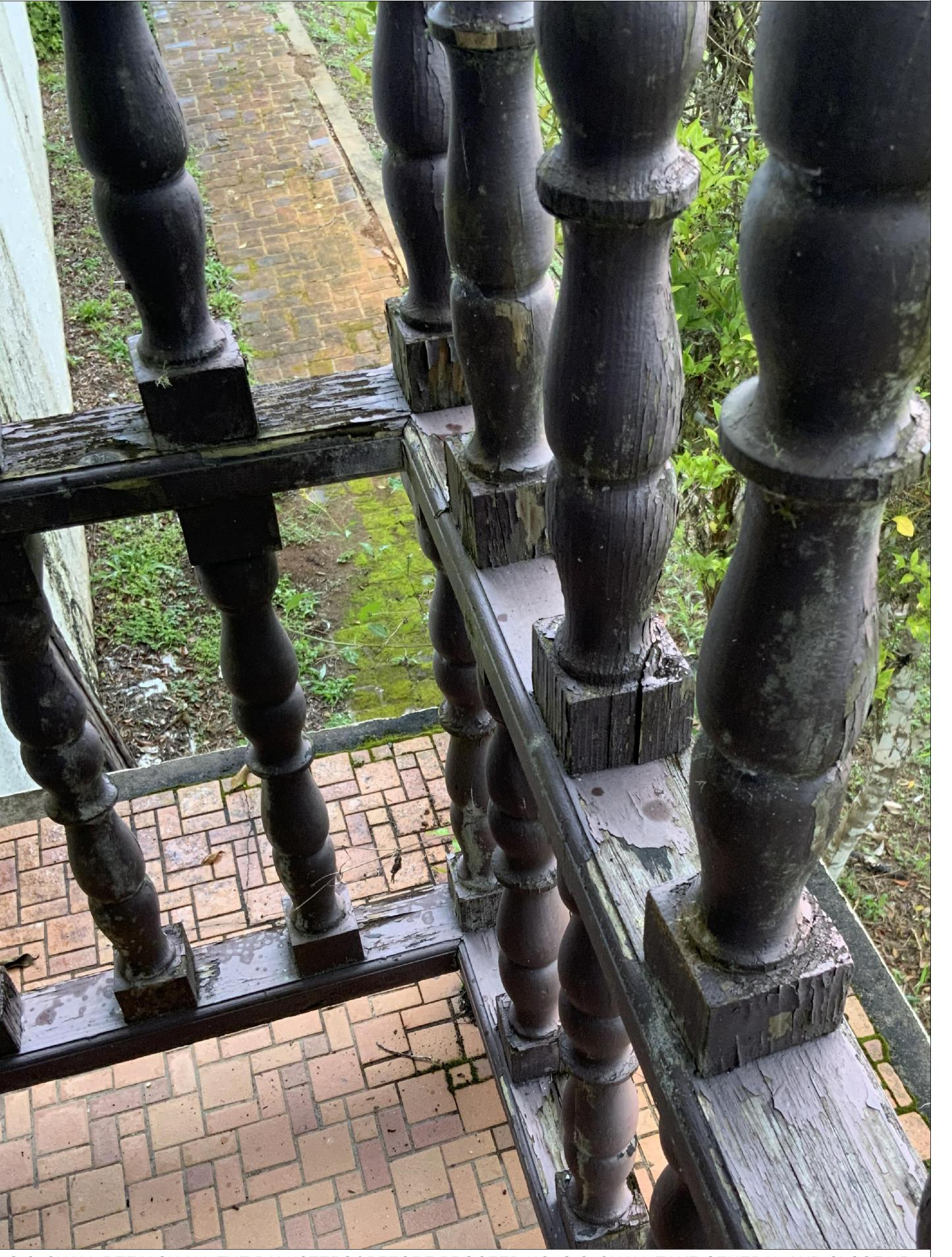
G.C. SHALL REFINISH ALL THE BALUSTERS | BEFORE PROCEEDING, G.C. SHALL TAKE GENERAL AND CLOSE UP IMAGES OF BALUSTERS CURRENT CONDITIONS FOR A/E REVIEW. | ENTIRE RAILING SHALL BE THOROUGHLY SCRAPPED FROM EXISTING PAINT BEFORE REPAINTING. | SEE FINISH NOTES FOR ADDITIONAL INFORMATION. | THIS REPAIR BELONGS TO ALTERNATE B.
