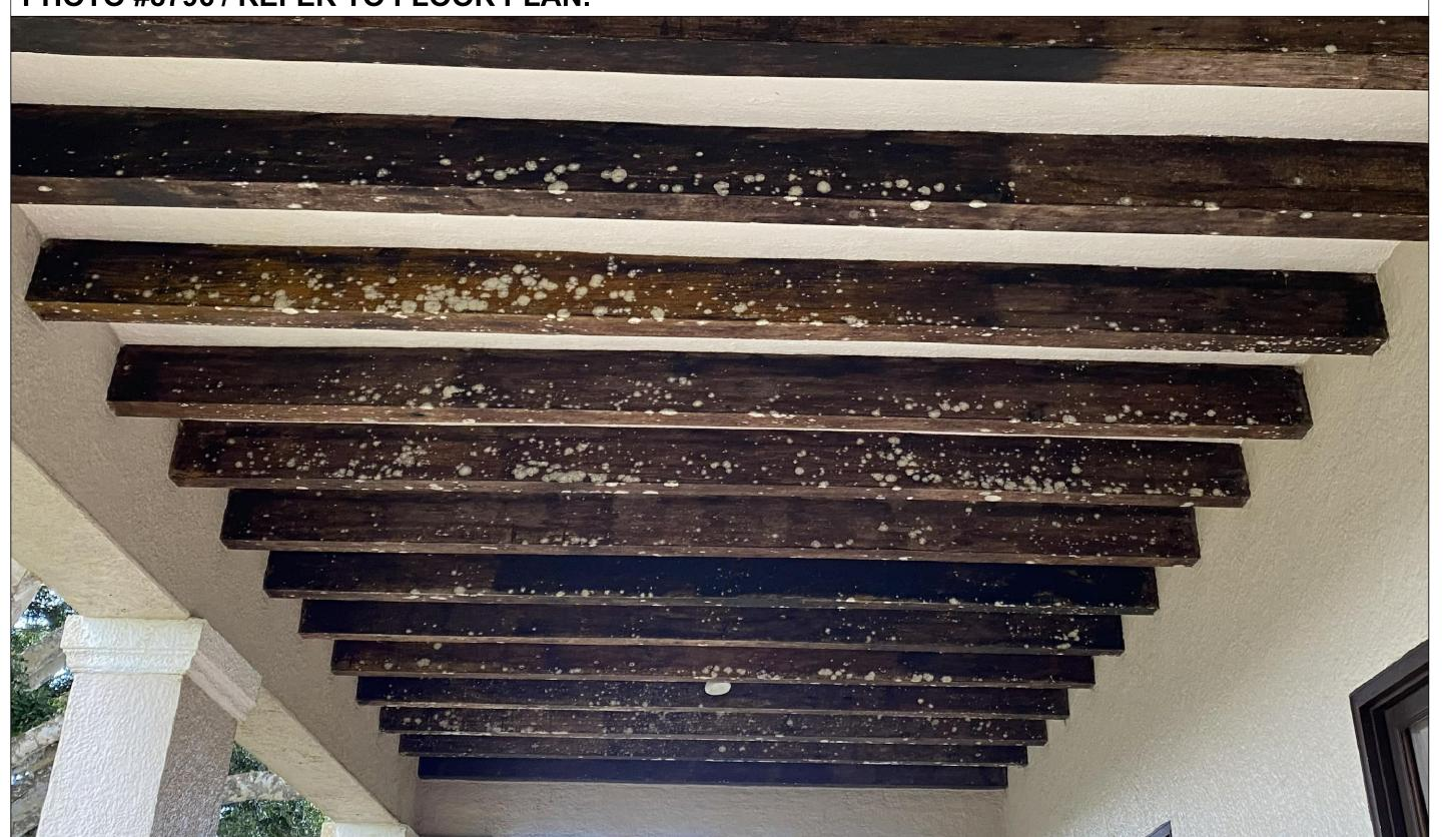
GENERAL CONTRACTOR SHALL THOROUGHLY DEEP CLEAN EXTERIOR WOOD BEAMS WITH PRESSURED WATER IN ORDER TO PROPERLY REMOVE ALL THE DIRT AND MOLD. SPECIAL CARE SHALL BE TAKEN WHEN USING PRESSURED WATER SO AS TO NOT DAMAGE THE BEAMS.
