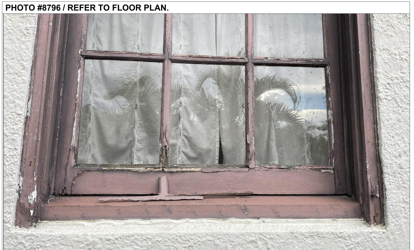
GENERAL CONTRACTOR SHALL REMOVE AND REPLACE EXISTING WOOD WINDOW MKD "H" WITH NEW ON SERVICE ROOM. | WINDOW CURTAINS SHALL BE REMOVED, CLEANED, STORED AND REINSTALLED. | SEE WINDOW DETAILS, SCHEDULE AND NOTES FOR ADDITIONAL IMPORTANT INFORMATION.
