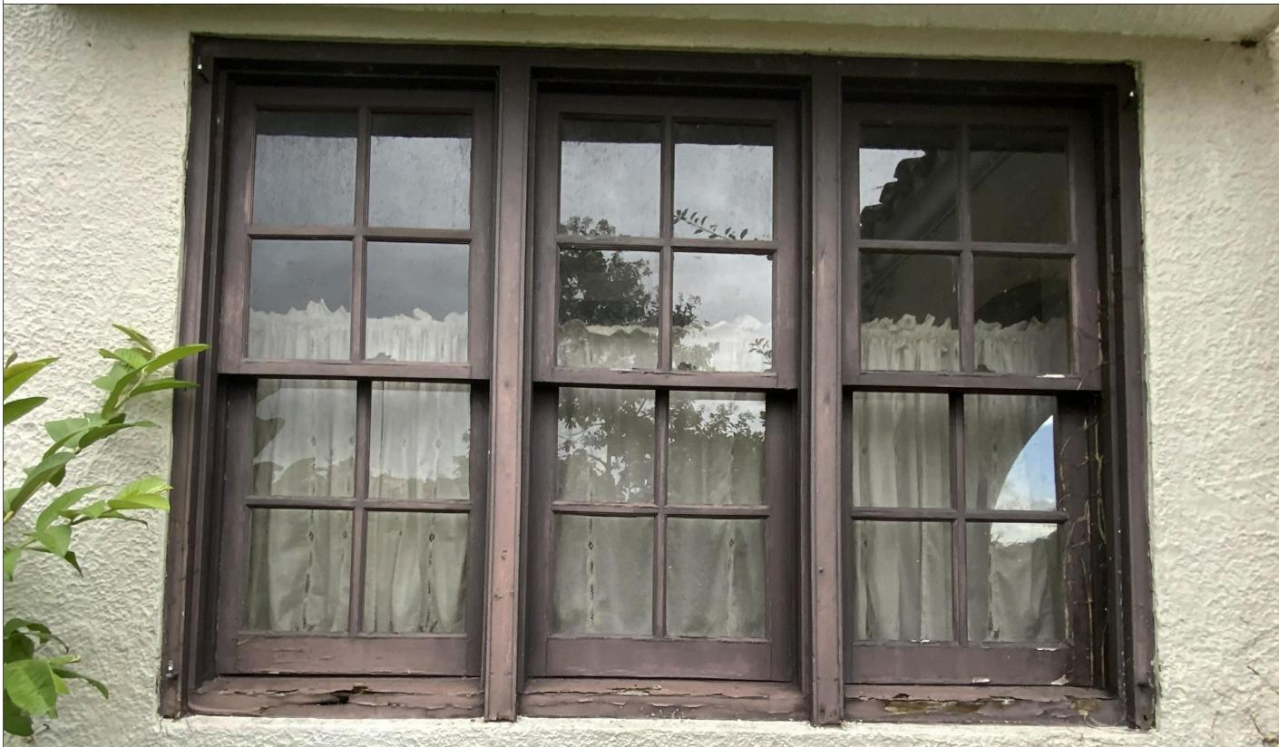
GENERAL CONTRACTOR SHALL REMOVE AND REPLACE EXISTING SINGLE HUNG WOOD WINDOW ON KITCHEN MKD "G" WITH NEW. | WINDOW CURTAINS SHALL BE REMOVED, CLEANED, STORED AND REINSTALLED. | SEE WINDOW DETAILS, SCHEDULE AND NOTES FOR ADDITIONAL IMPORTANT INFORMATION. SEAL ALL PERIMETER.
