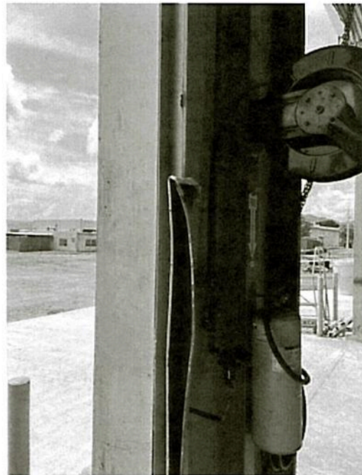
Image 8. Damage guides on Bldg 1052
