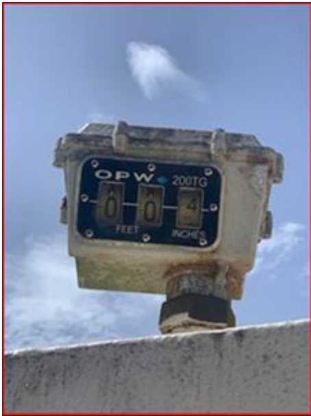
Figure 24. Mechanical Level Gage
