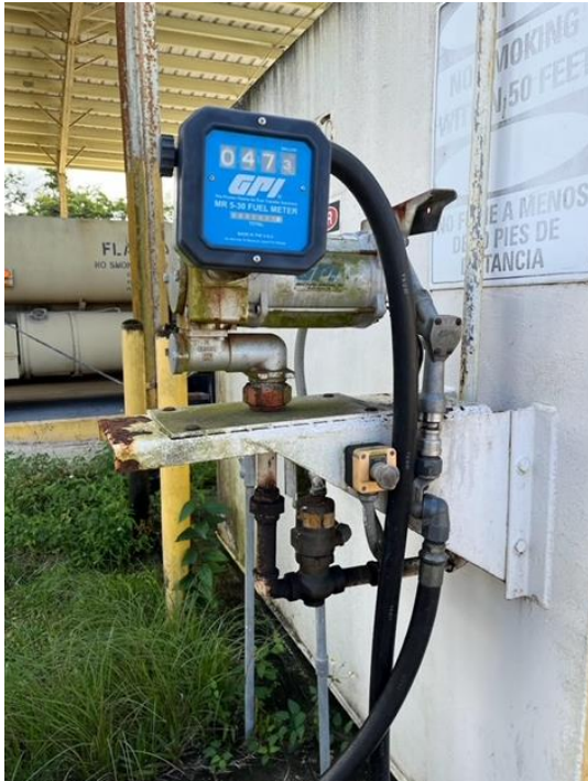
Figure 7. Dispenser and flow meter system (GPI)
