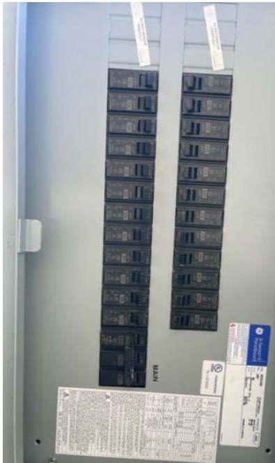
Figure 30. Breakers Main Panel Board
