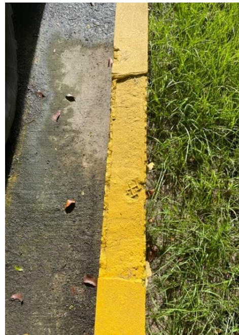
Figure 19. Left side broken edges of Spill Control Area
