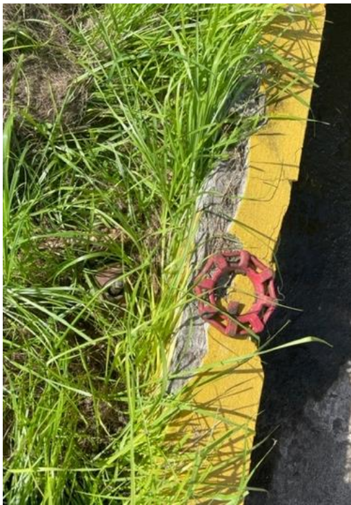
Figure 18. Broken Gate Valve
