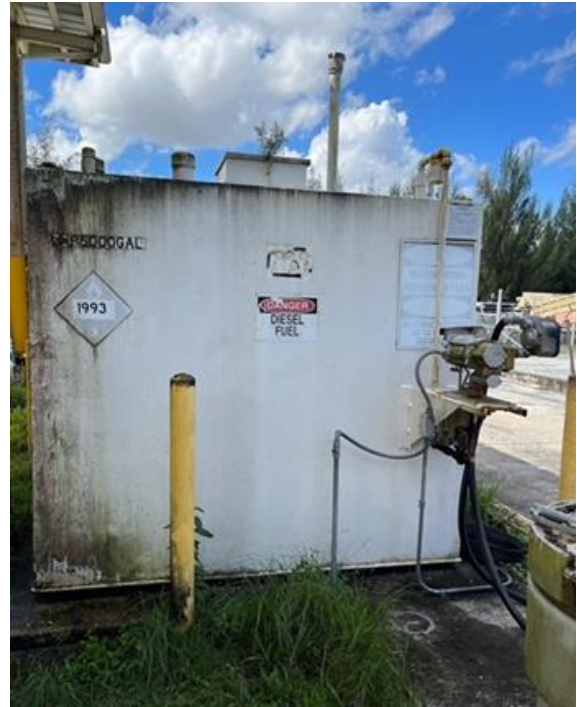
Figure 2. Left View of Above Storage Tank (Capacity: 5,000 Gal)
