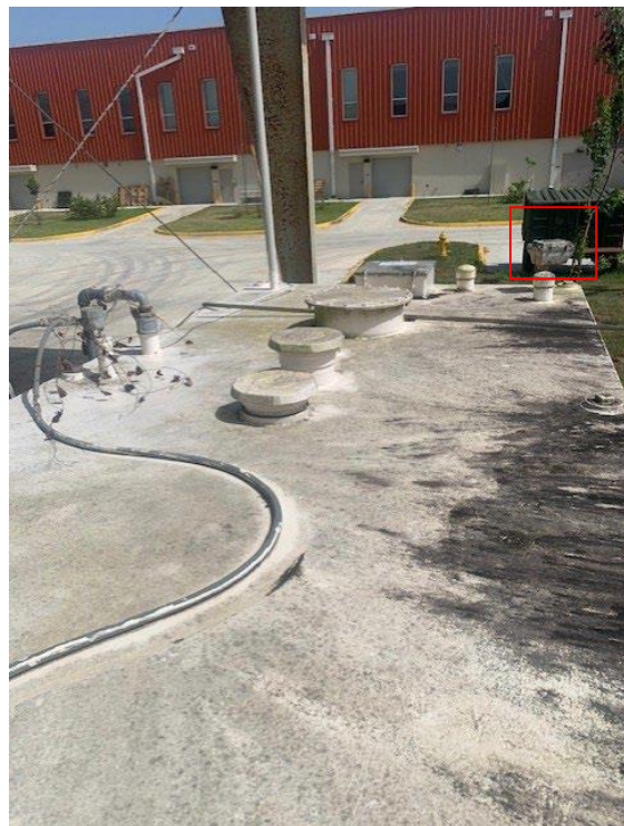
Figure 23. Top View (Vents, Manholes &amp; fittings)
